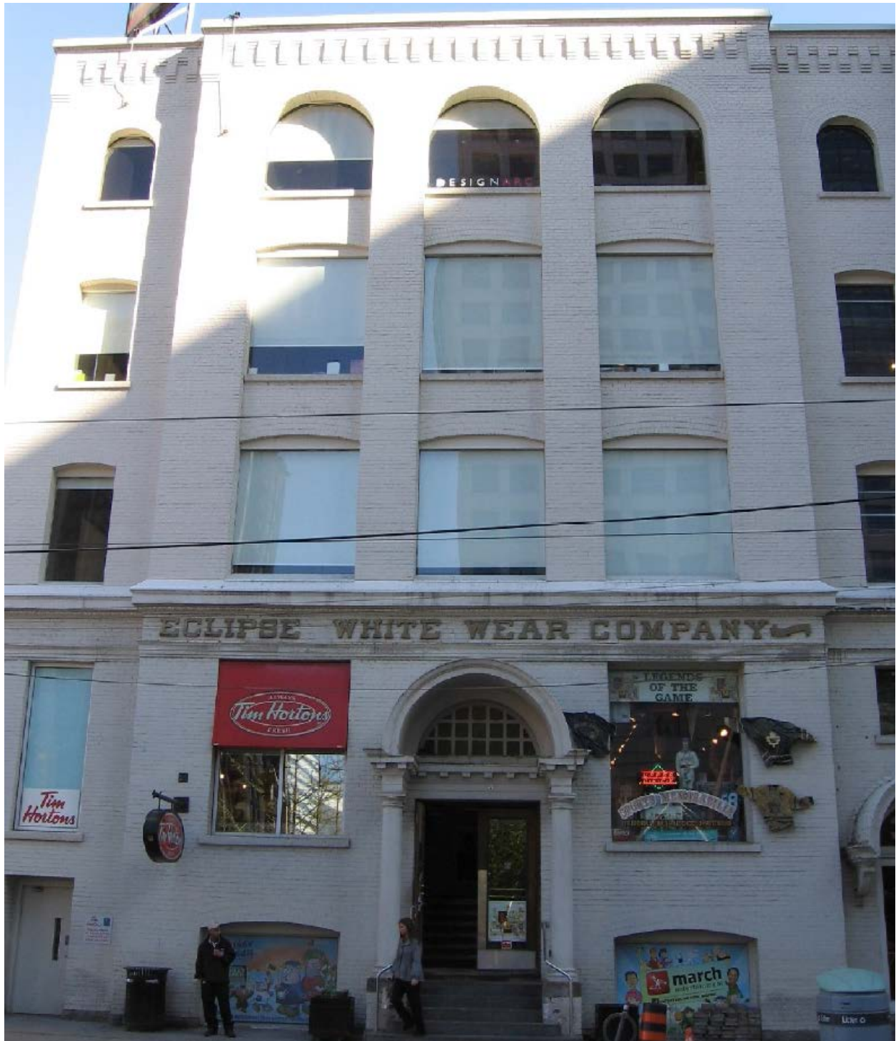
322 King Street West - Eclipse Building
