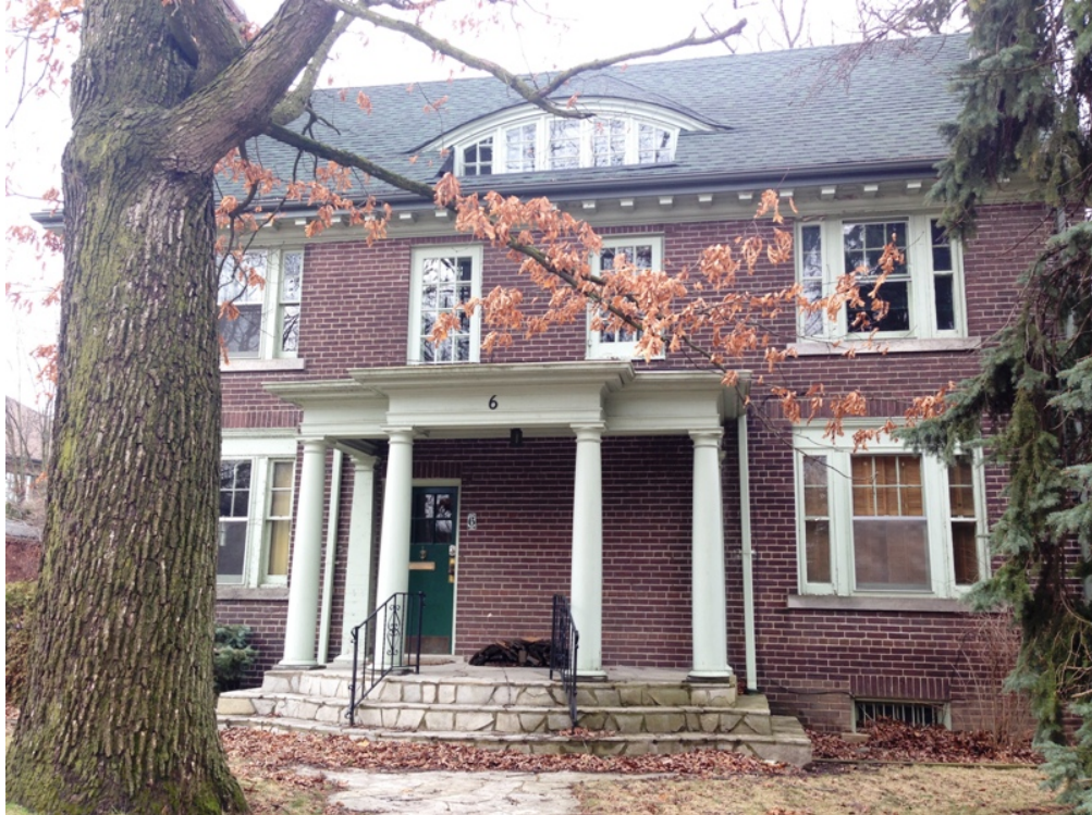
15. 6 Frank Crescent, principal (east) elevation with the arrangement of main entry door and the portico. (HPS, 2017)
