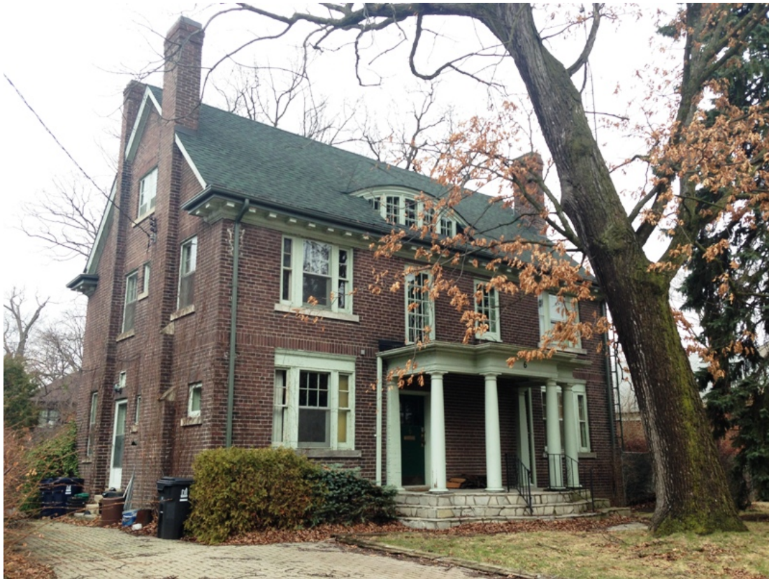
14. 6 Frank Crescent, principal (east) and side (south) elevations (HPS, 2017)
