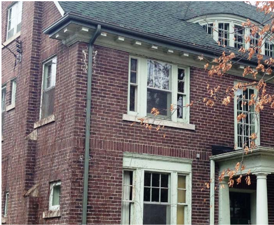
18. 6 Frank Crescent, details including the portico column and pilaster capitals and entablature, the window frames, stone sills, brick belt course of headers, tapering chimney with stone caps, cornice with return eaves, mouldings and mutules on the underside of the eaves, attic dormer and mouldings (HPS, 2017)
