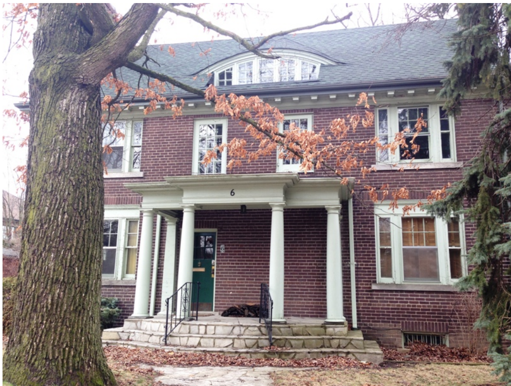
6 Frank Crescent: looking towards the south (side) and east (principal) elevations (above) and at the east elevation (below) (Heritage Preservation Services [HPS], 2017)
