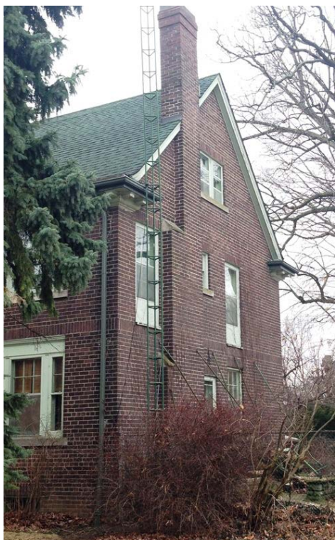
16. 6 Frank Crescent, the north (side) elevation including second floor door openings to the demolished verandah (HPS, 2017)
