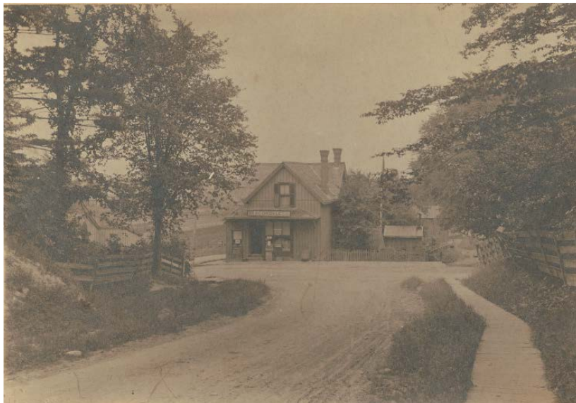
6. Bracondale Post Office, at the south-west corner of Christie and Davenport Road. Taken between 1898 and 1910. (CTA, Fonds 2, Series 8, File 40, Item 1)
