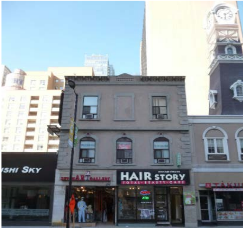
480 Yonge Street facade - west side of the block
