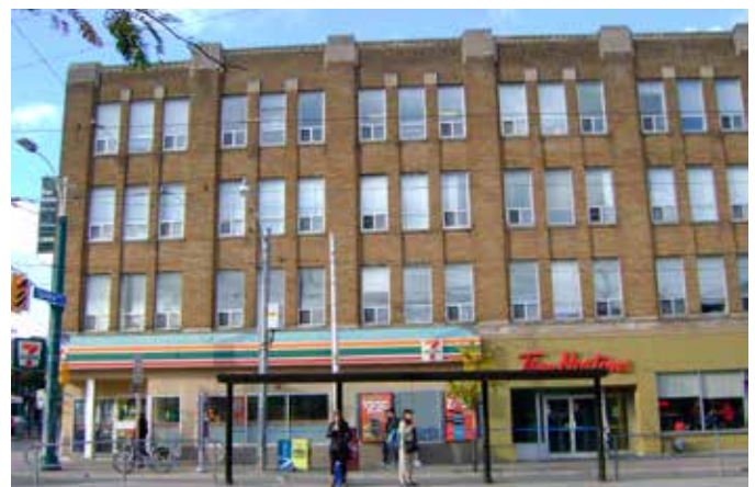
Loft style commercial building
