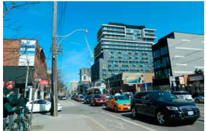
Recent development on College Street
