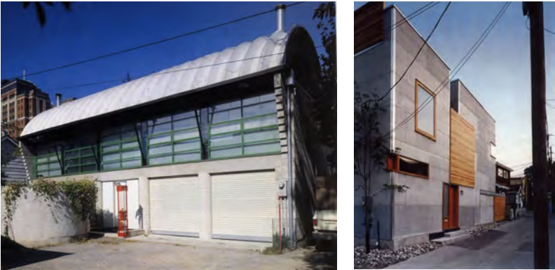
Stinson house – credit Jeffery Stinson + Terence Van Elslander Existing Toronto laneway houses show precedent for residential life on laneways and surmounting servicing and access issues, but are generally much greater in scale than the proposed as-of-right permitting process would allow
