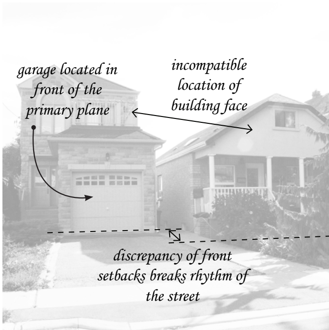
Figure 47 Incompatible building face
