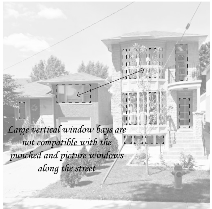
Figure 63 Incompatible window size and spacing
