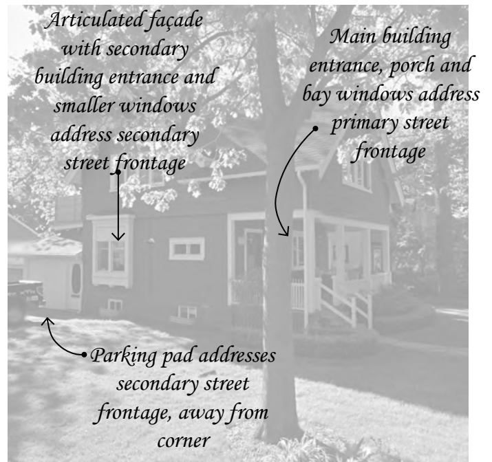
Figure 108 Designed and articulated to address both street frontages in an equally enhanced manner
