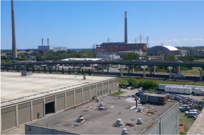
View towards the Hearn Stack from within the Precinct
