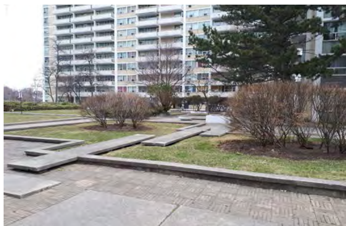
Figure 2.16: Decommissioned fountain feature in open courtyard at 45 Oakmount Road.
