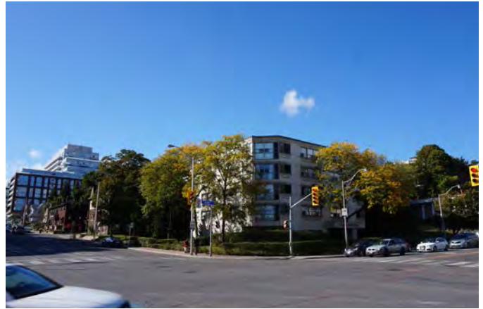
Figure 2.30: The tall apartment buildings of the study area disappear from view at a local topographical low point near the south-east corner of Bloor Street West and Keele Street.
