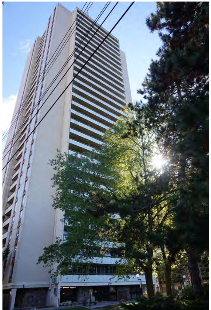
Figure 2.40: Tower in the Park era point tower apartment building.
