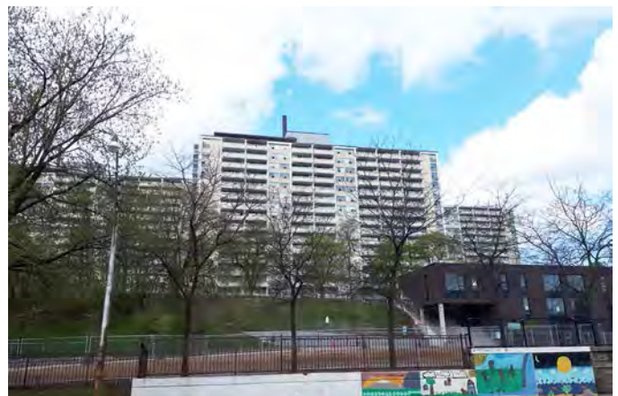
Figure 1.2: Apartment buildings within the study area visible beyond Keele Street Public School grounds.
