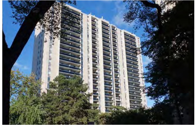
Figure 2.39: Tower in the Park era slab-form apartment building.
