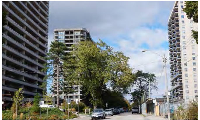
Figure 3.38: Tower separation across a street within the study area.
