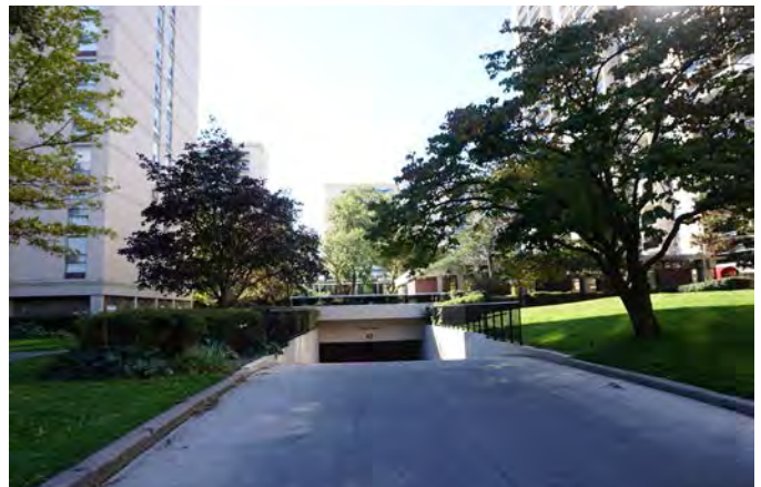
Figure 2.21: Free-standing, underground parking access ramp.
