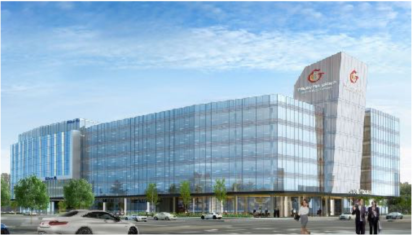
Figure 5 - VIEW OF PROJECT FROM SOUTHEAST
