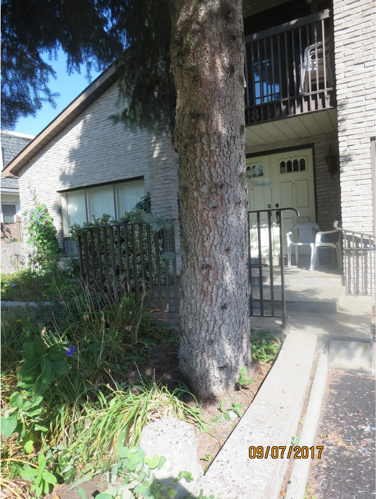
Attachment 2: Photograph showing the base of the tree in relation to the east retaining wall.
