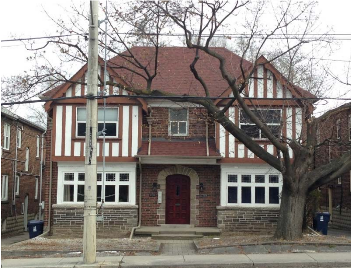
18. 1767-1769 Bayview Avenue (HPS, 2017)
