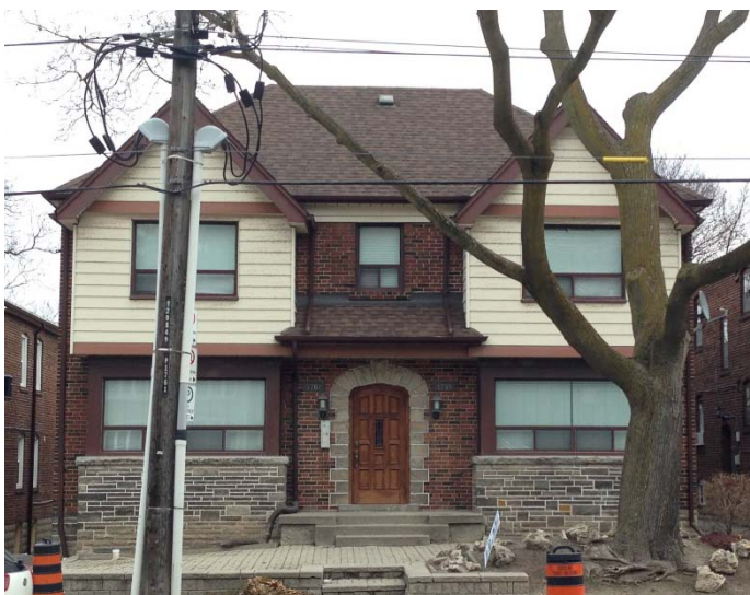
16. 1759-1761 Bayview Avenue (HPS, 2017)
