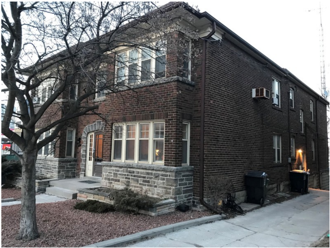
10. 1783-1785 Bayview Avenue, north and west elevations (HPS, 2018)
