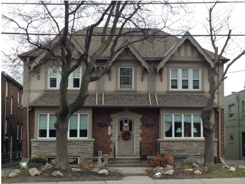
13. 1747-1749 Bayview Avenue (HPS, 2017)
