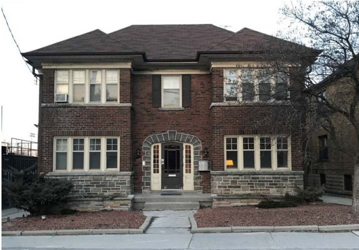
Photograph of the principal (west) elevation at 1783-1785 Bayview Avenue (Heritage Preservation Services (HPS), 2018)
