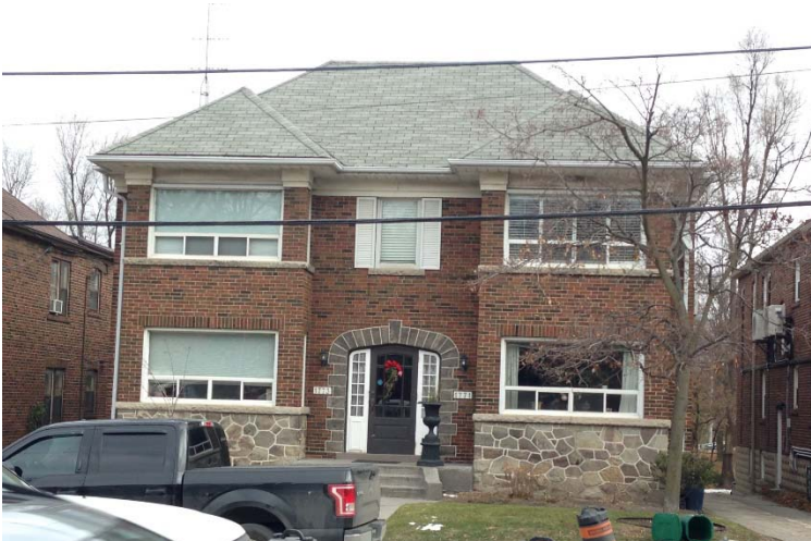
19. 1771-1773 Bayview Avenue (HPS, 2017)
