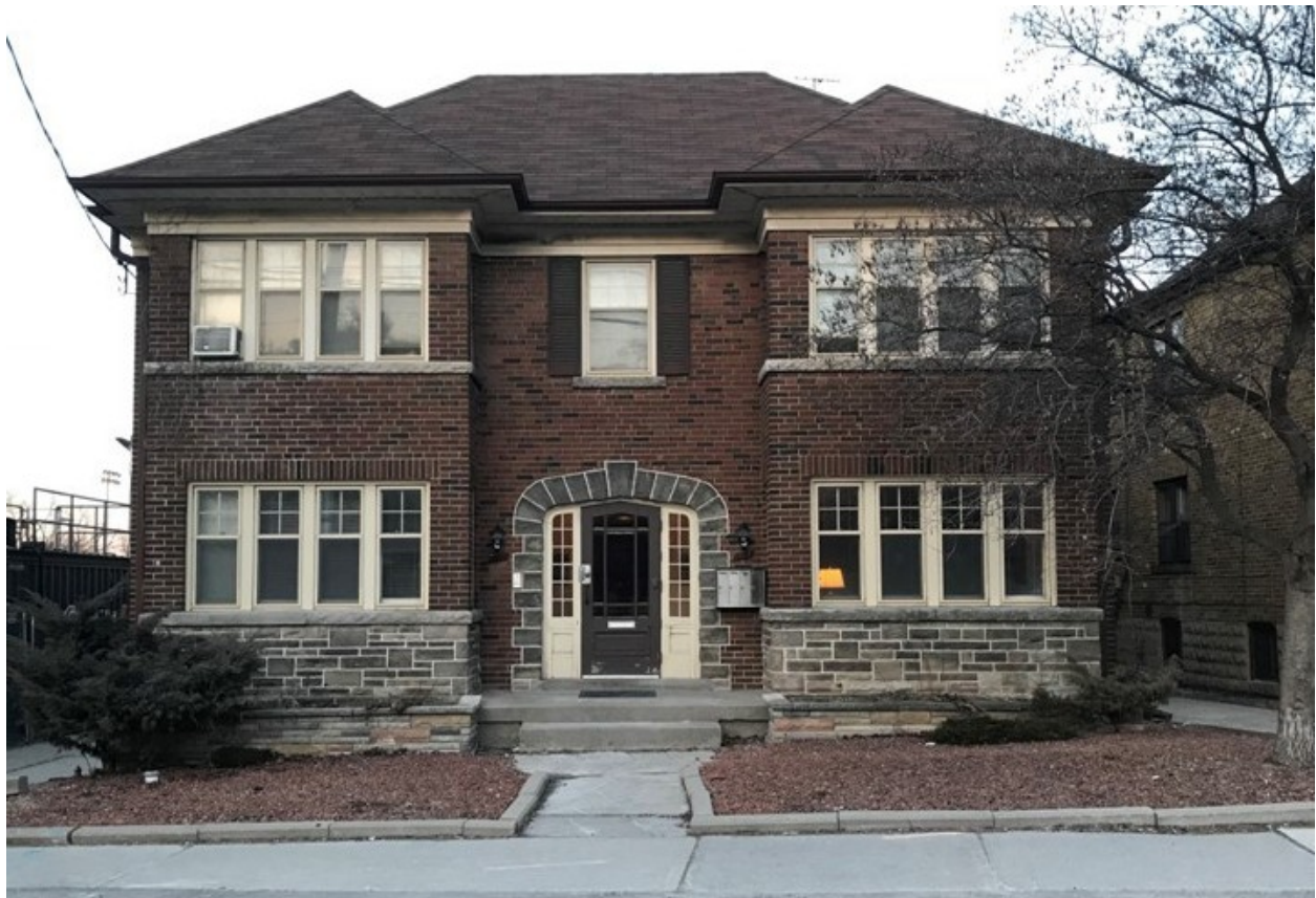
9. 1783-1785 Bayview Avenue, principal (west) elevation (HPS, 2018)
