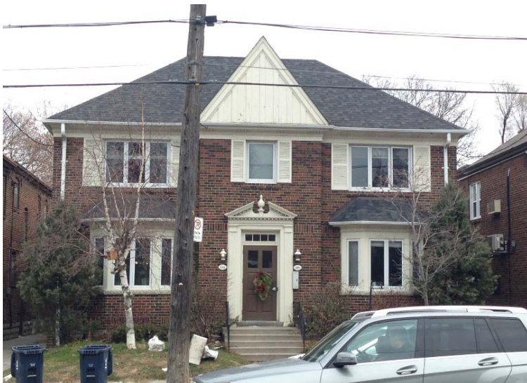
14. 1751-1753 Bayview Avenue (HPS, 2017)
