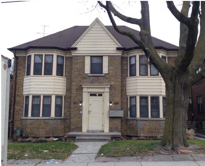
21. 1779-1781 Bayview Avenue (HPS, 2017)
