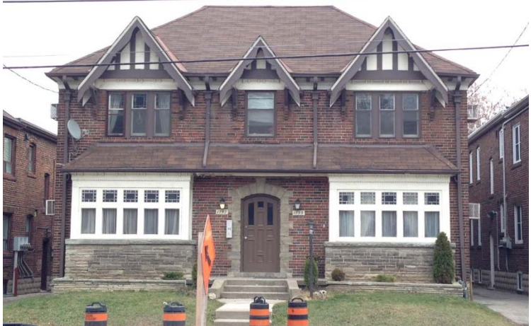
15. 1755-1757 Bayview Avenue (HPS, 2017)
