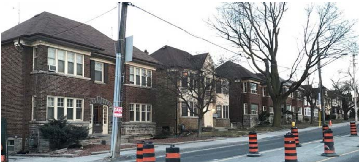
Photograph looking south on the east side of Bayview from 1783-1785 Bayview Avenue showing the set of 10 apartment buildings and their similarity in massing and variety in style. (HPS, 2018)
