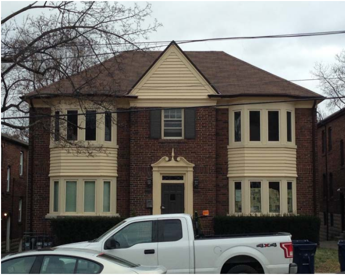
17. 1763-1765 Bayview Avenue (HPS, 2017)
