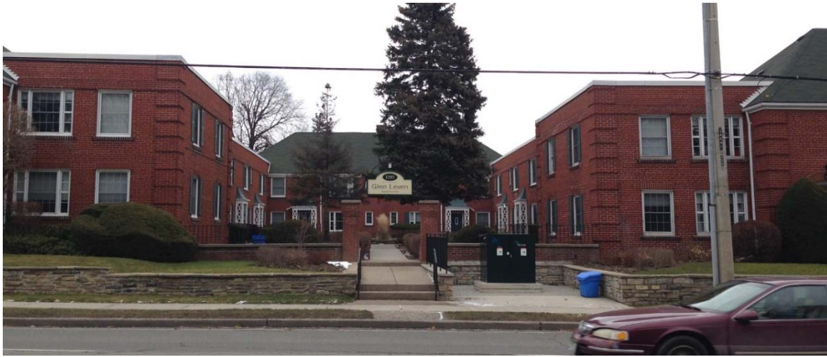
26. Glen Leven apartments at 1365 Bayview Avenue, also constructed by Talbot and representing consistent scale and period as well as demonstrating variety of housing types (HPS, 2017)
