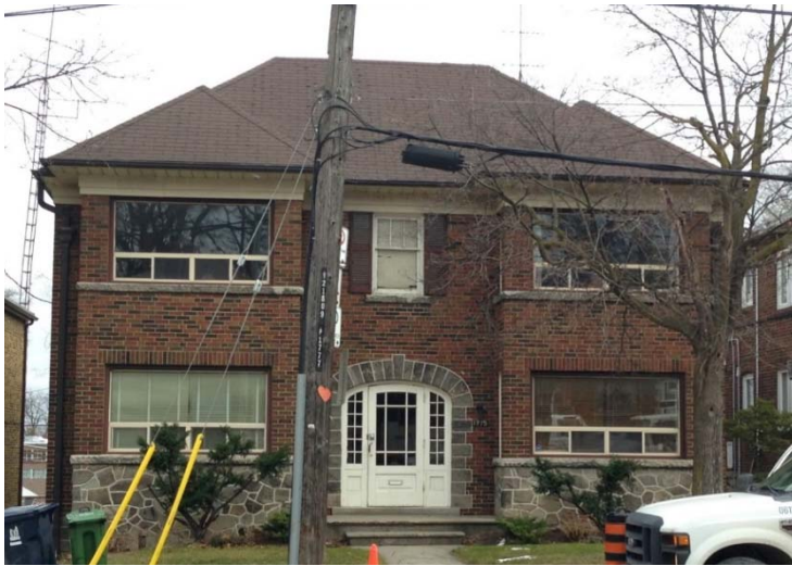
20. 1775-1777 Bayview Avenue (HPS, 2017)
