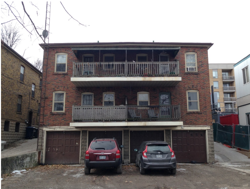
12. Rear (east) elevations of 1783-1785 Bayview Avenue showing the balconies and integrated garages. (HPS, 2017)
