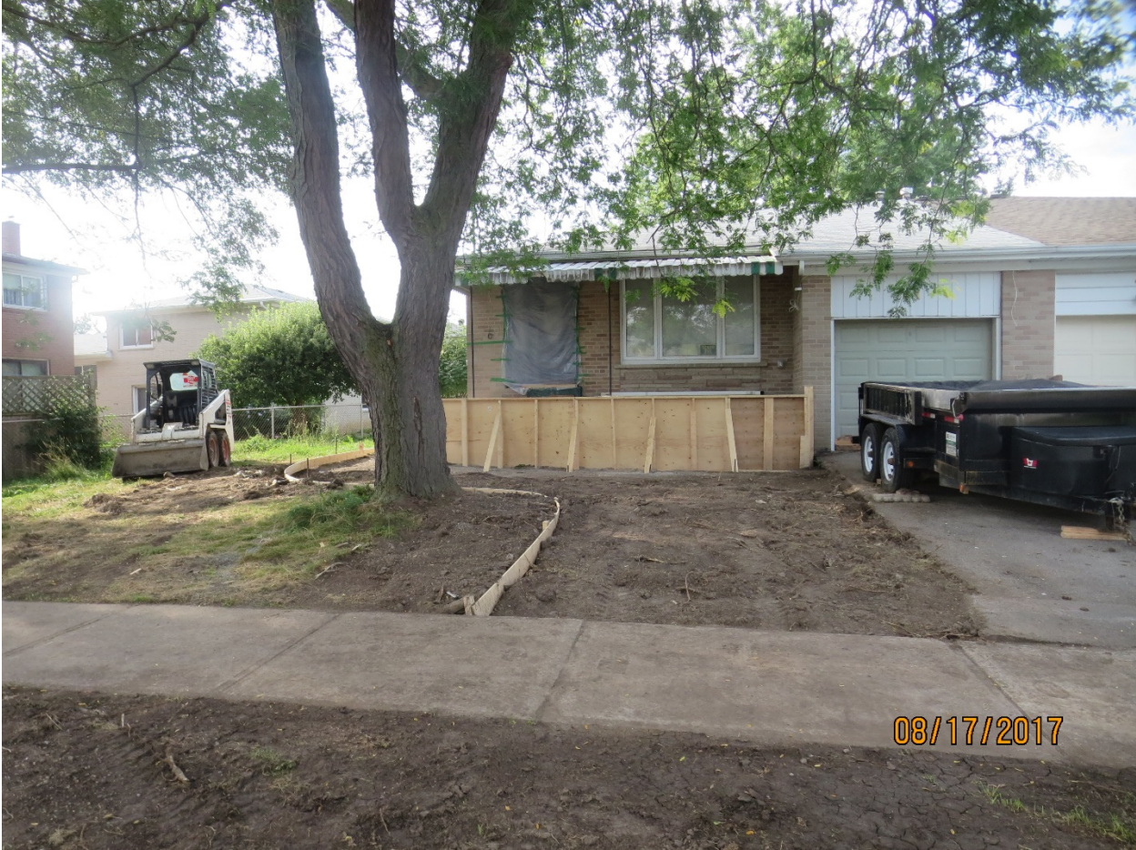
Attachment 2: Photograph of the August 2017 tree bylaw contravention with excavation and compaction within the tree protection zone of the honey locust tree
