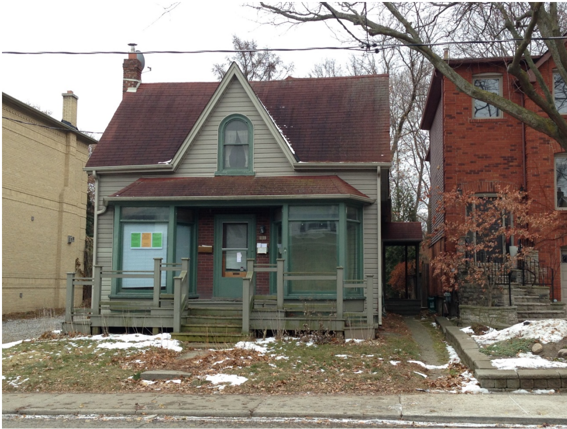
8. 505 Balliol Street, principal (north) elevation (HPS, 2017)
