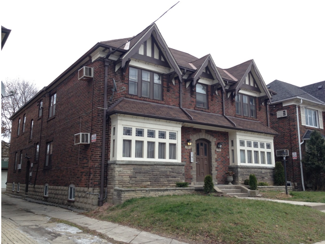
11. 1755 Bayview Avenue, north and west elevations (HPS, 2017)
