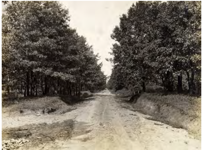
Figure 23: Construction of Baby Point Road
