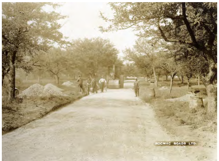
Figure 24: Construction of Baby Point Road (2)
