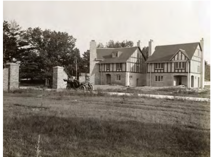
Figure 22: Construction of homes at Baby Point, 1913
