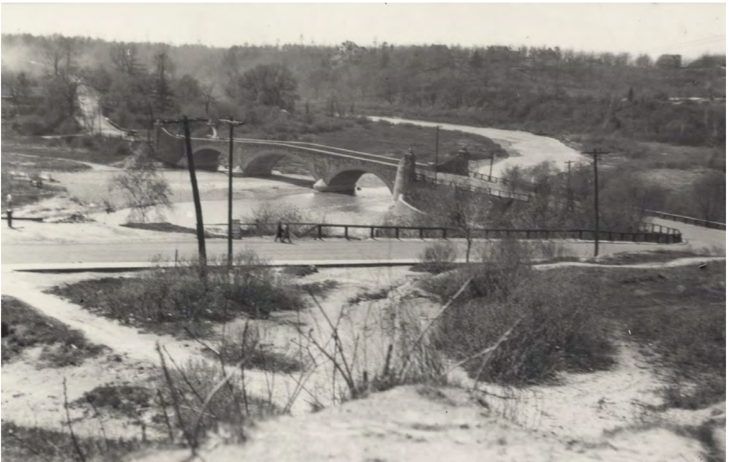
Figure 27: Old Mill Rd., looking west to bridge (built 1916) across Humber River. Viewed between Catherine Street & Old Mill Road
