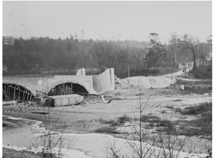
Figure 26: Old Mill Road looking west showing the bridge across the Humber River and Gamble mill, 1918
