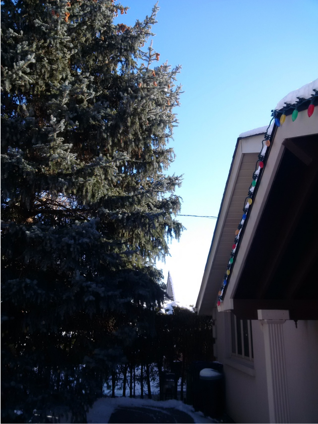
Attachment 2: Photograph showing the clearance distance between the house located at 34 Cartier Crescent and the blue spruce measuring 41 cm in diameter
