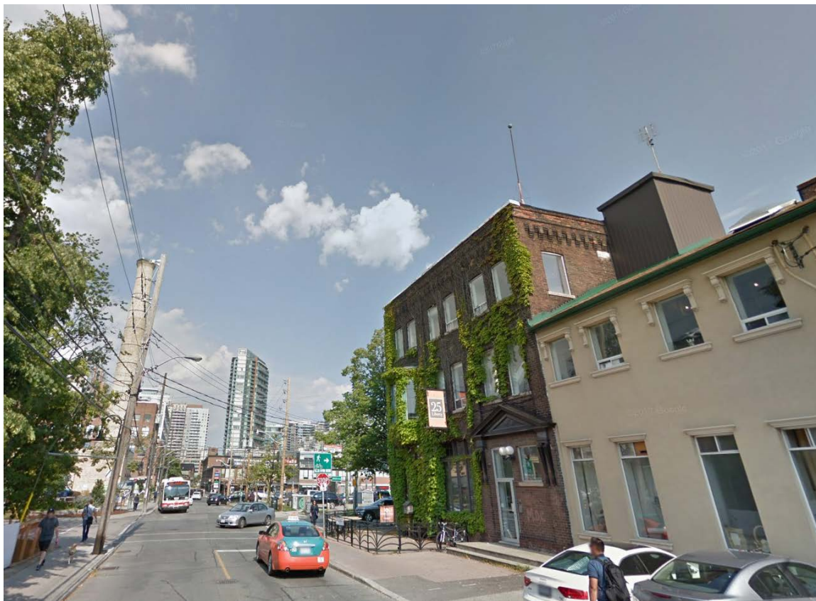
View of development site looking east along Liberty Street
