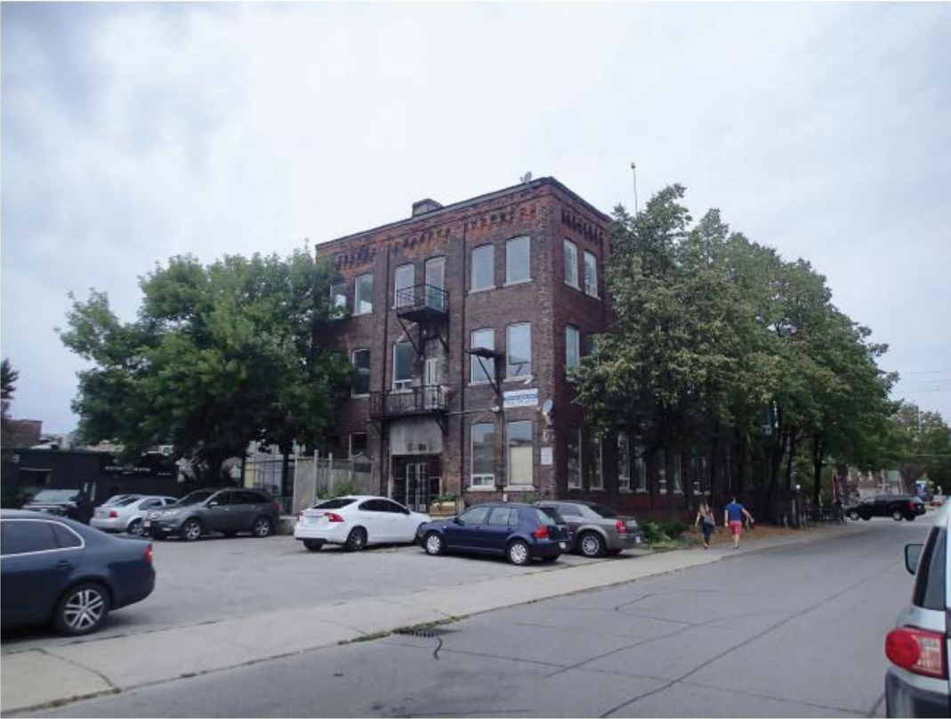
View of development site: south and east elevations looking northwest from Atlantic Avenue
