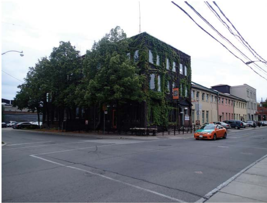
View of development site: east and north elevations looking south west from Liberty Street and Atlantic Avenue
