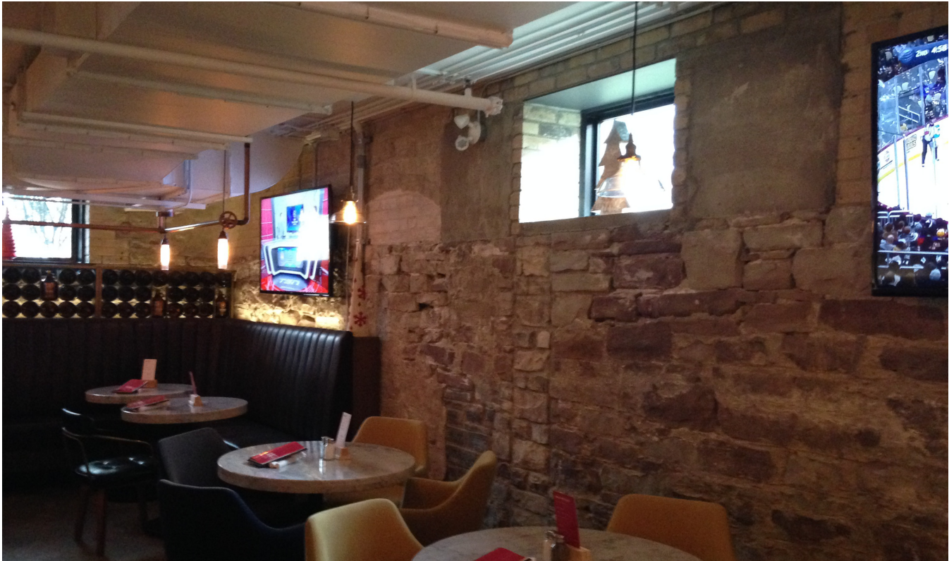
Figure 6: Photo of south basement wall of 60 Atlantic along Liberty Street, directly north across Liberty Street from the Ontario Wind Engine and Pump Company Building. The original brick and stone rubble foundation has been preserved, exposed and utilized as a successful heritage element within the Big Rock Brewery restaurant.
