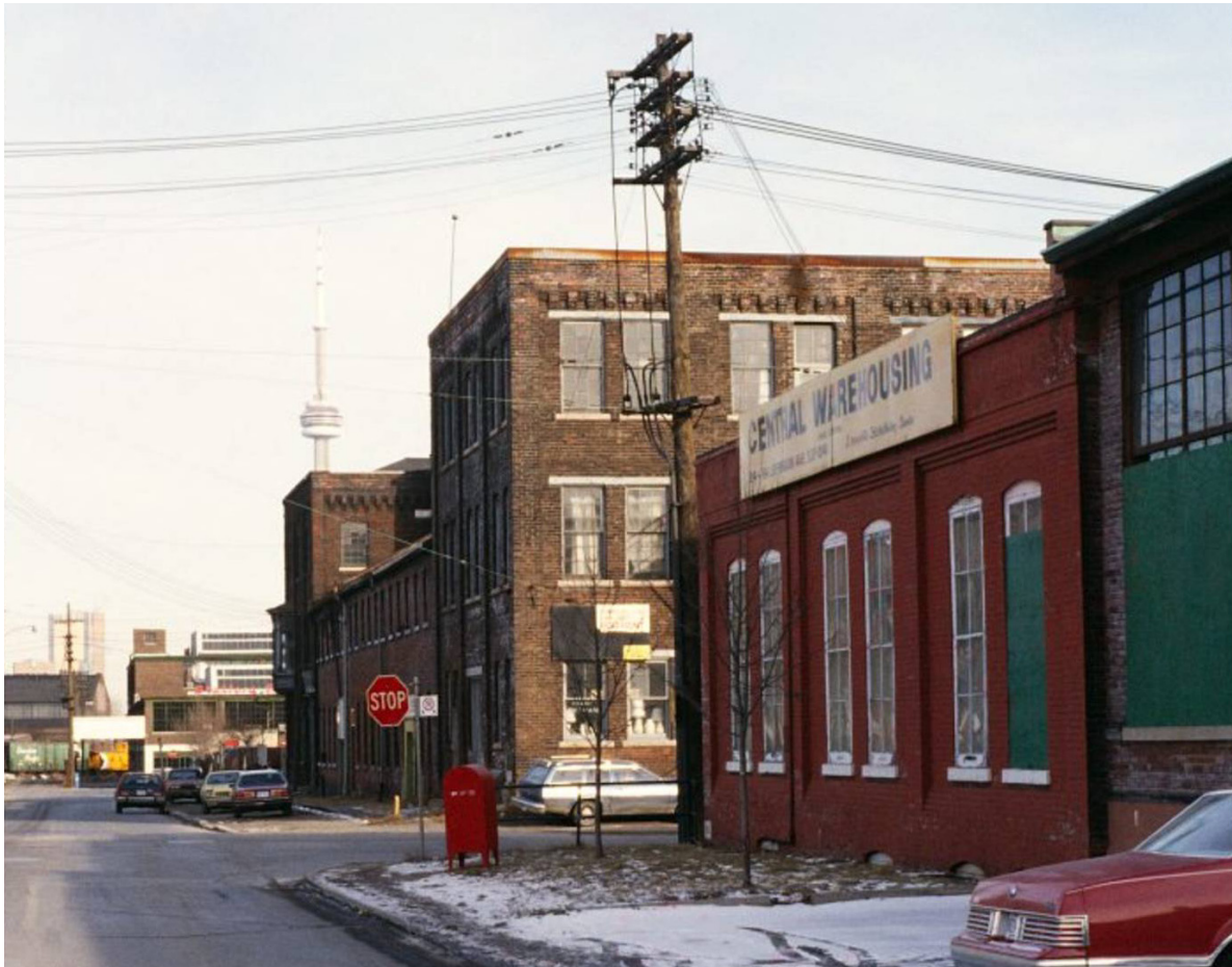
Figure 1: Photo looking east along Liberty Street at Jefferson Ave, c.1980s with all original brick facades intact on 35 Liberty and 65 Jefferson Ave.
