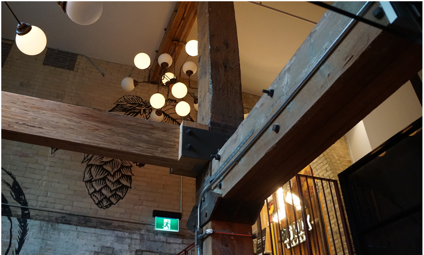
Figure 8: Exposed original post-and-beam framing at the Big Rock Brewery restaurant inside 60 Atlantic, across Liberty Street from the Ontario Wind Engine and Pump Company Building.
