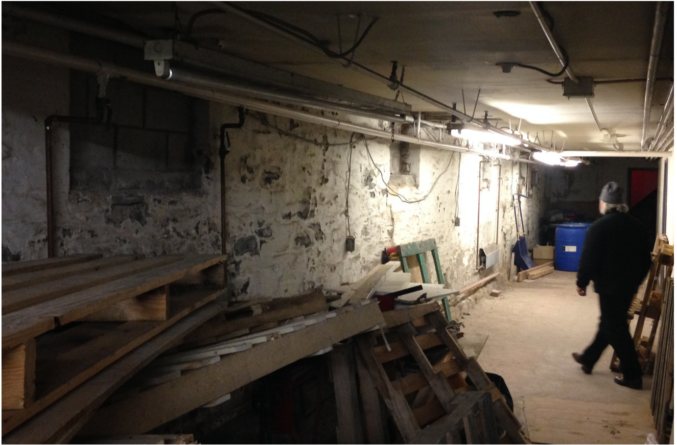
Figure 5: Photo of north basement foundation wall of 35 Liberty along Liberty Street indicating original stone rubble foundation wall. The basement under 35 Liberty Street also contains original fireproof brick arch ceilings and tin counterweight fire doors throughout the basement level.
