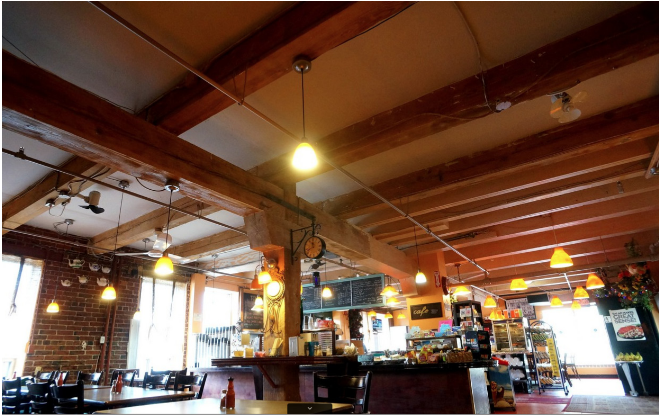
Figure 7: South view inside the ground floor of the Liberty Village Market and Cafe at 65 Jefferson Ave showing the exposed post-and-beam framing. This framing continues intact throughout the upper 2 floors of the building. The original post-and-beam framing is also intact throughout 35 Liberty Street.
