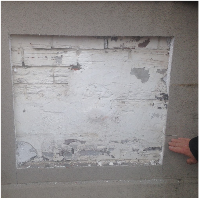
Figure 4: Enlarged details of west facade of 65 Jefferson Ave. with approx. 20" x 20" section of recently removed stucco finish on Styrofoam insulation layer exposing the original brick masonry wall.
