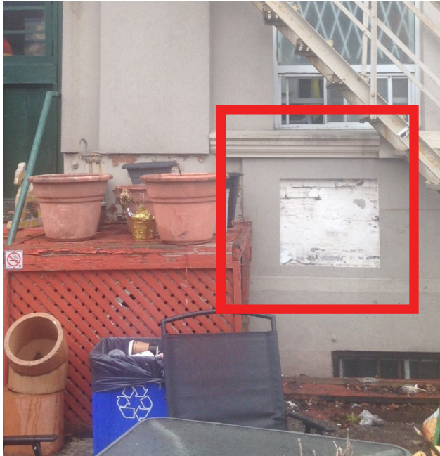
Figure 4: Enlarged details of west facade of 65 Jefferson Ave. with approx. 20" x 20" section of recently removed stucco finish on Styrofoam insulation layer exposing the original brick masonry wall.
