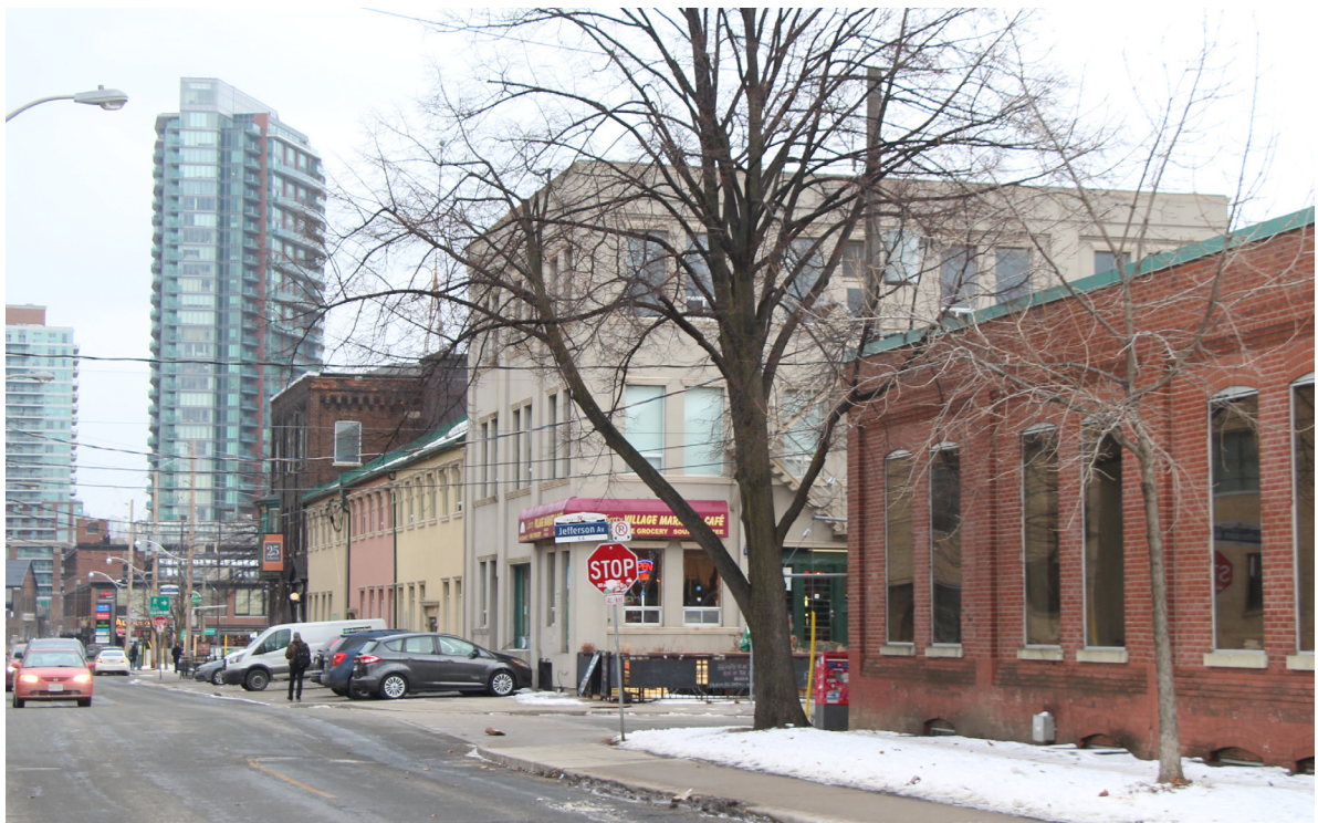
Figure 2: Same vantage point, February 2018 showing 65 Jefferson and 35 Liberty street with a stucco exterior facade.
