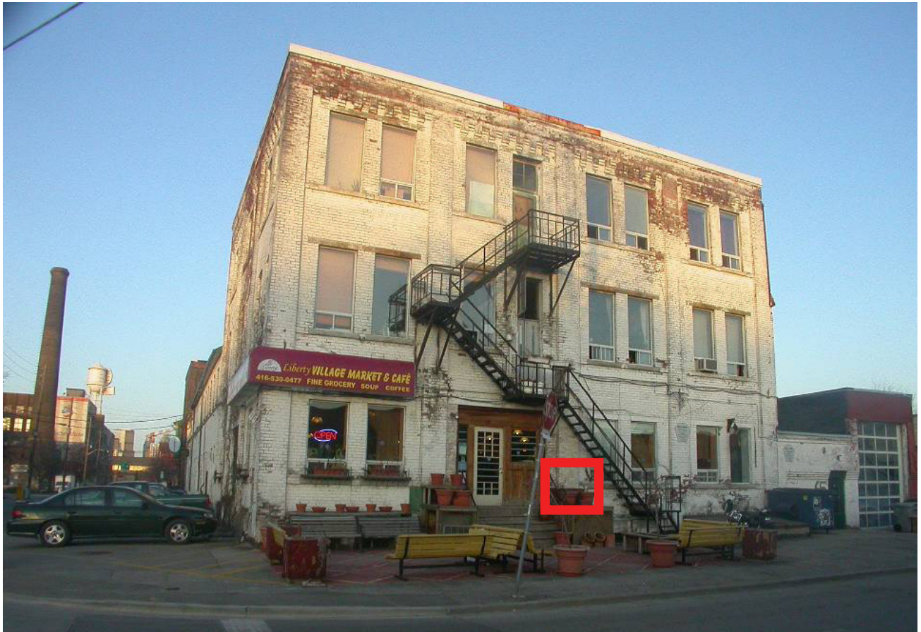
Figure 3: Photo looking east at the corner of Liberty Street at Jefferson Ave, c.1990s. The brick facade of 65 Jefferson Ave. and 35 Liberty Street are painted white. Red rectangle indicates area of recently revealed original brick facade visible below stucco and Styrofoam insulation.
