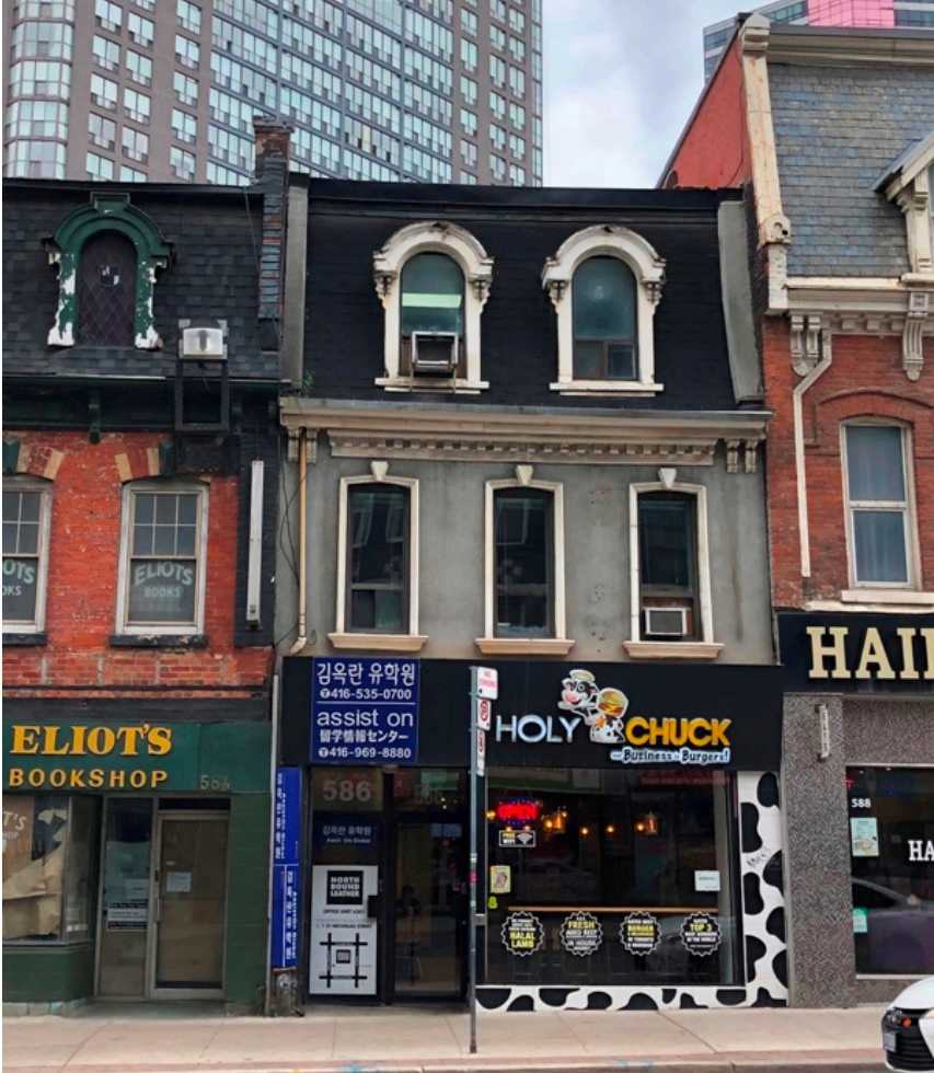
Photograph of the principal (east) elevation of 586 Yonge Street (HPS, 2019)
