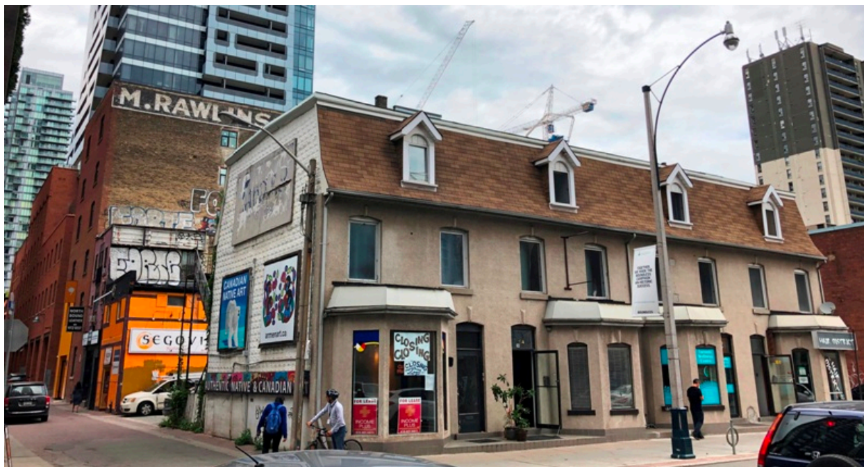
Photograph of 10-16 Wellesley Street West at the north-east corner with St. Nicholas Street showing the principal (south) and side (west) elevations and the properties at 5-7 St. Nicholas Street to the left in the distance (Heritage Preservation Services [HPS], 2019)
