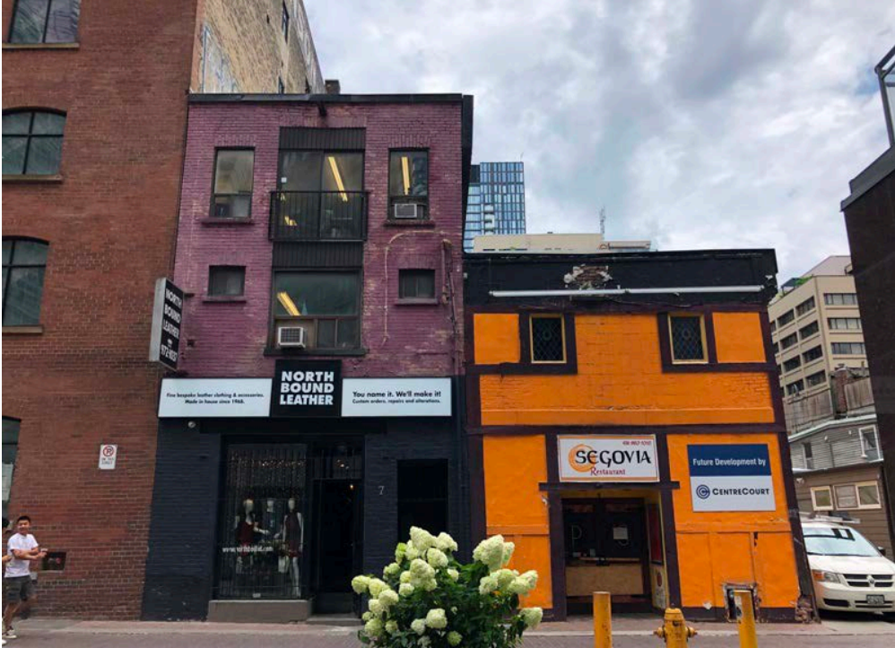
Photograph of the principal (west) elevations of 7 St. Nicholas Street and to the right, 5 St. Nicholas Street (HPS, 2019)
