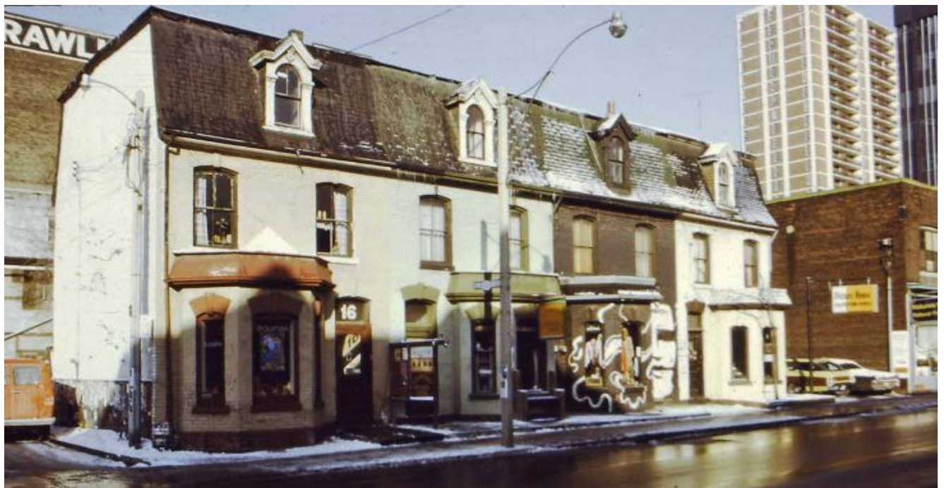
10. 1974 Archival photo of the row at 10-16 Wellesley Street West showing the original window sashes with the double hung two-over-two double hung sashes and the attic dormers (CTA, Toronto Historical Board Fonds 2043, series 2523)
