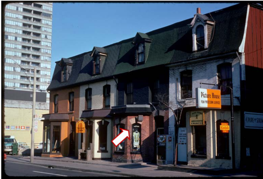
9. 1975 Archival photo of 10-16 Wellesley Street West showing the restored brick at No. 12 with the yellow brick headers over the window and door openings. (CTA, Harvey R. Naylor, fonds 1526, File 2, Item 56, 1975)
