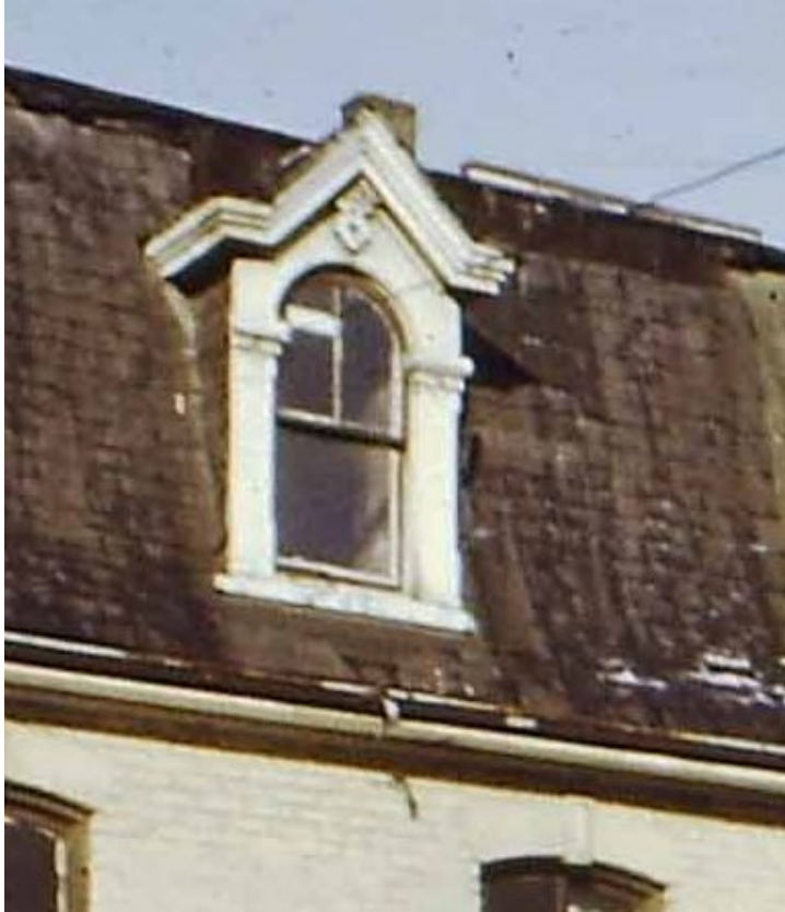
11. Enlarged detail of the above photo to show the details of the dormer roof, gable and the wood piers (CTA, Toronto Historical Board Fonds 2043, series 2523)
