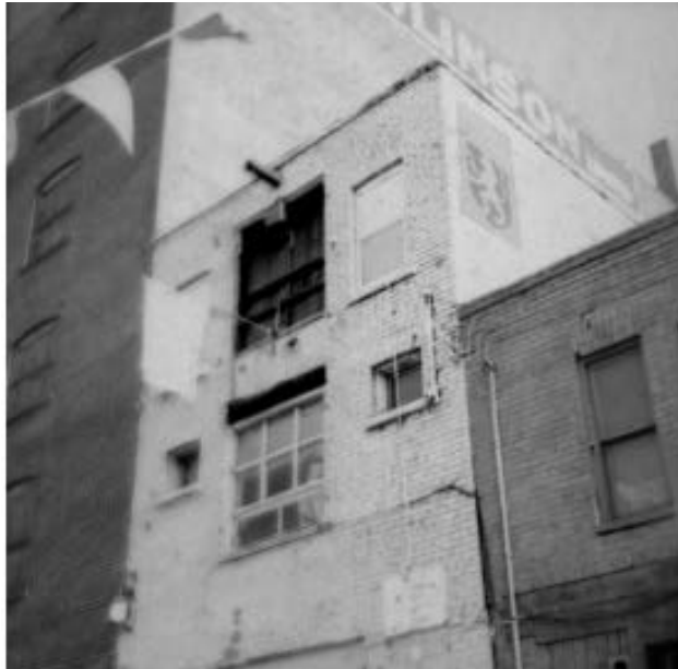
16. View of 5-7 St. Nicholas Street showing No. 7 during its occupation by the Bohemian Embassy (1960-1966) and the condition of the central openings before they were renovated and the original window opening at 5 St. Nicholas Street before it was renovated and stained glass windows replaced the originals and the brick cladding was covered with stucco and half-timbering ( Behind the Bohemian Embassy )
