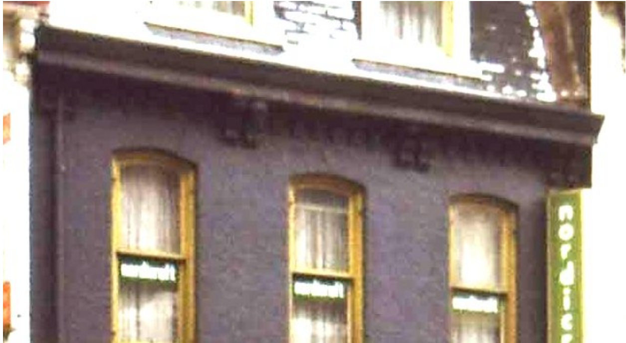
14. 586 Yonge Street, 1974, enhanced detail to show the original four pairs of brackets at the eaves and the corbels course in between with two-over-two double hung sash windows with curved heads and no keystones. (CTA, Toronto Historical Board Fonds 2043, series 2523)
