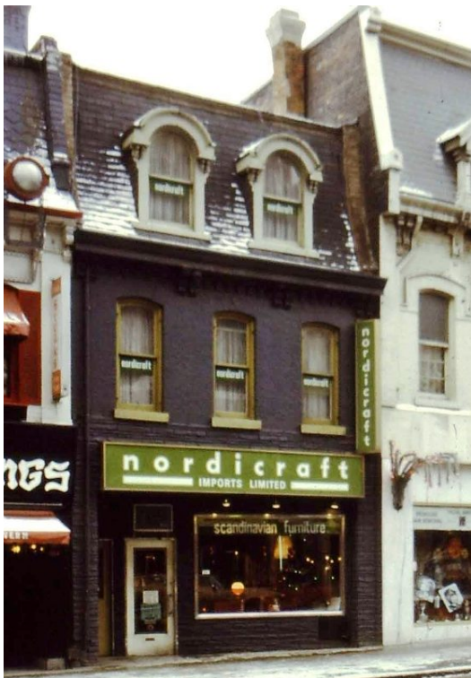
13. 586 Yonge Street, 1974 showing the original brick elevation at the upper level and the double hung sash in the dormers (CTA, Toronto Historical Board Fonds 2043, series 2523)
