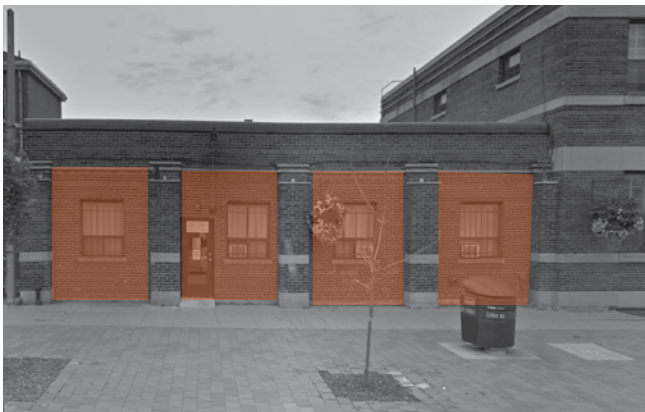
Fig. 19/ Existing photo, showing bricked in openings in orange
