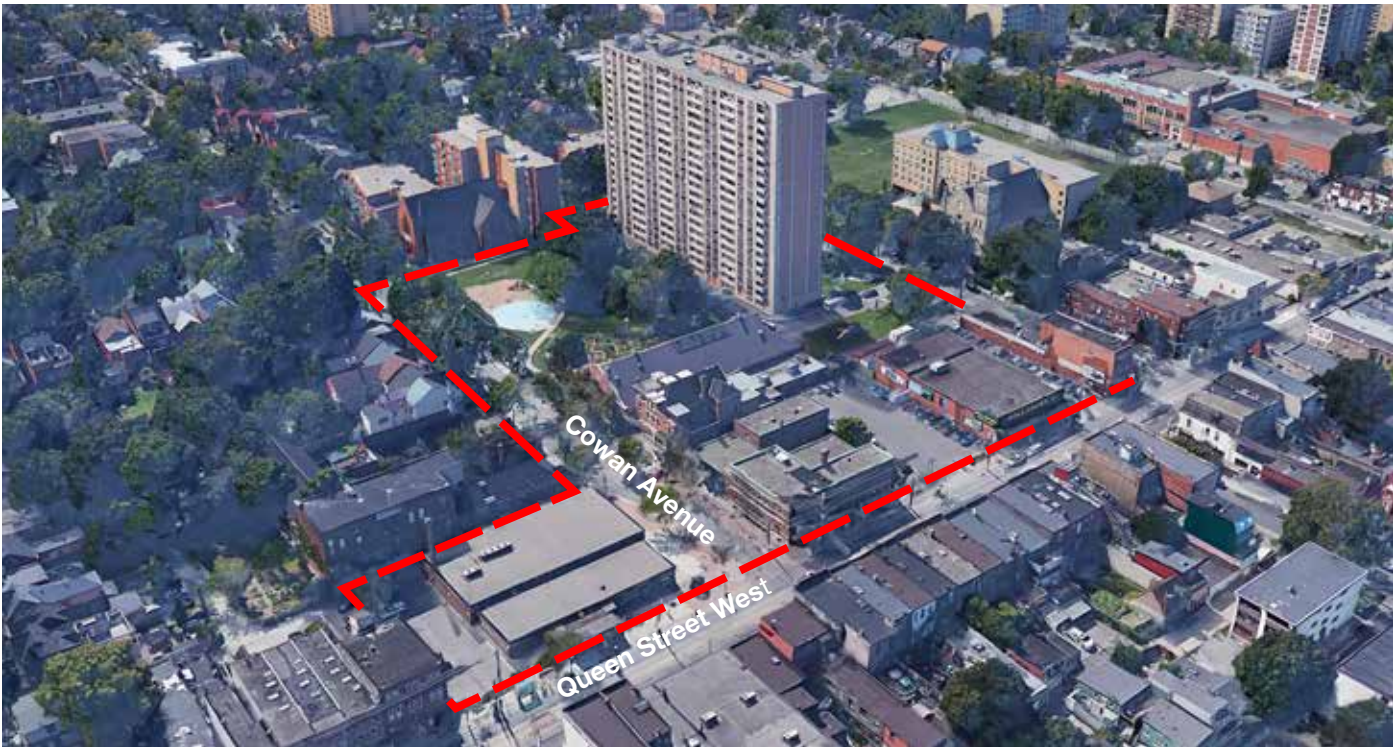
Fig. 3/ Aerial View Looking Southwest
