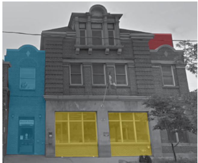
Fig.14/ Current photo of Fire Hall building, showing alterations
