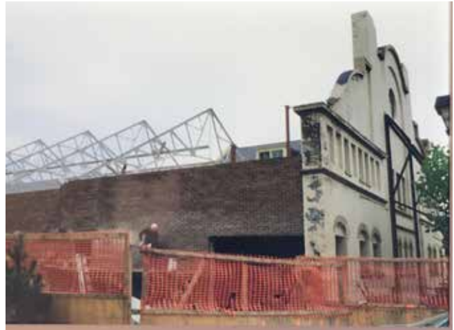
Fig.13/ Masaryk-Cowan Community Centre under construction, showing retention of front facade and trusses (Toronto Archives).
