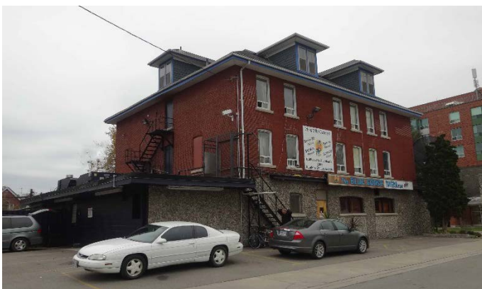
4c. north elevation on Manchester Street, facing the railway tracks (right), with the rear (east) elevation (left)
