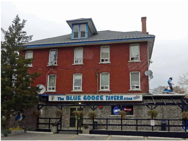
4a. west elevation on Blue Goose Street
