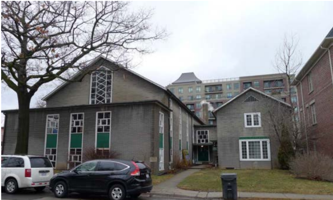
View (facing north) of the existing paved entry court on the east side of the church between the church, chapel/office building and rectory
