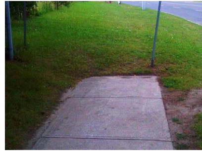
Missing Links Sidewalk Program
