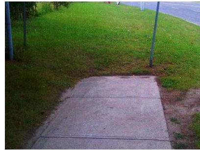
Missing Links Sidewalk Program
