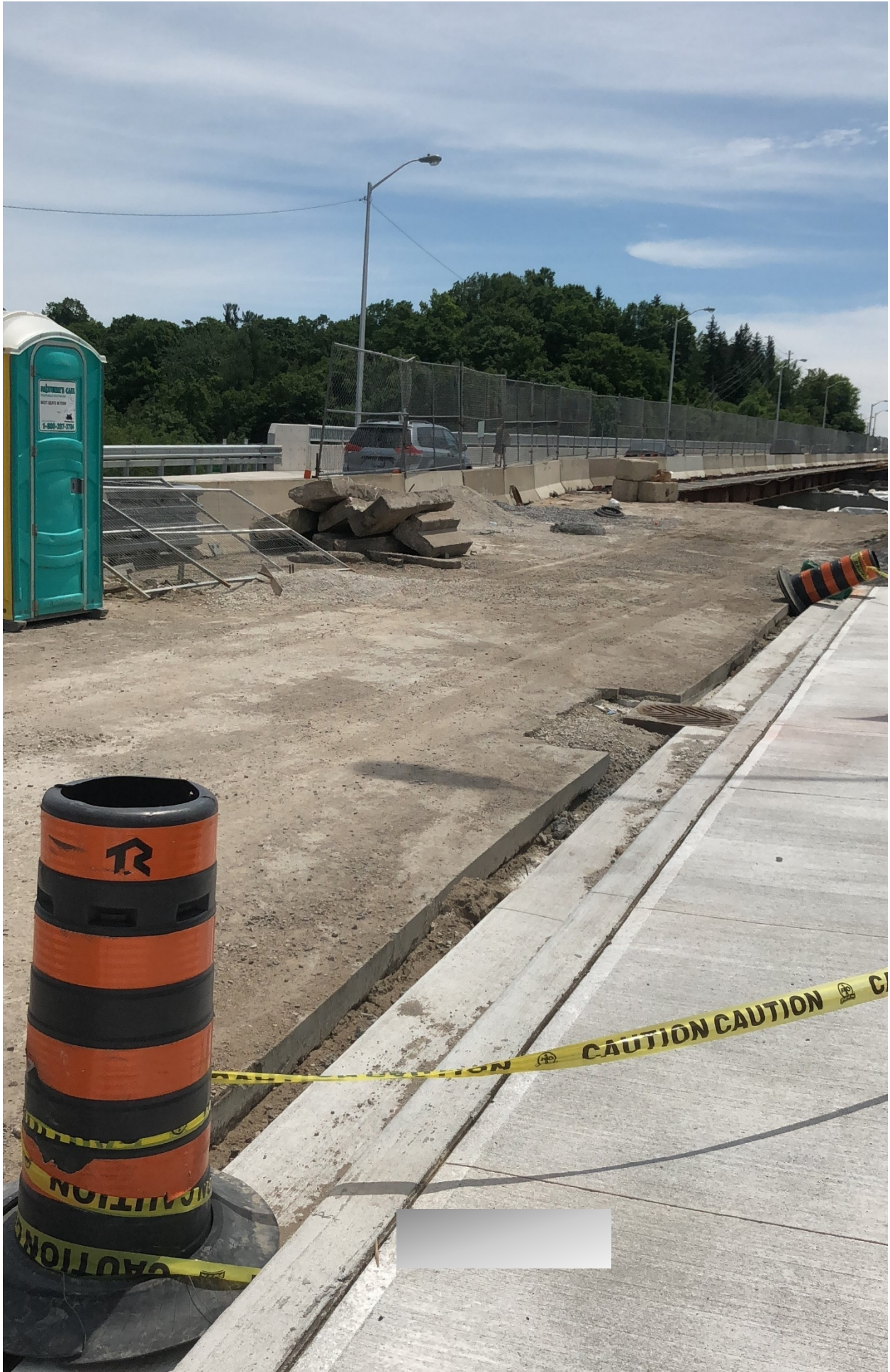
Attachment 7 – Unrestricted access to work zone and drop-off to valley below
