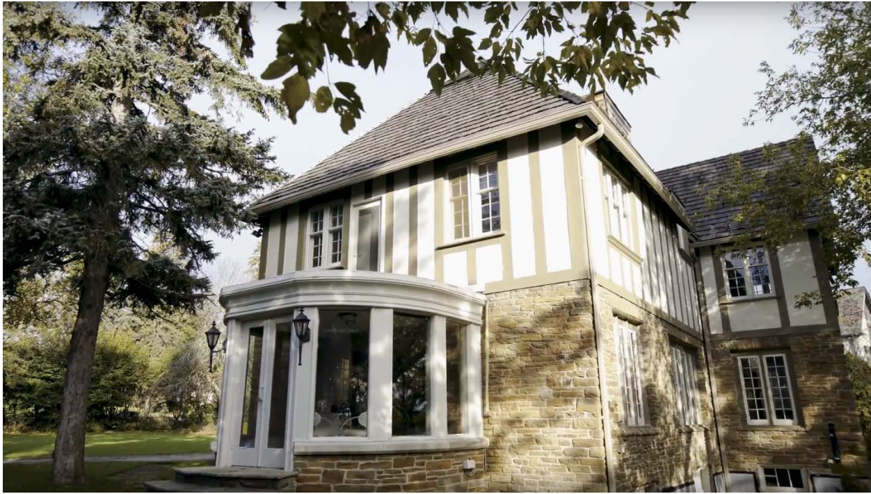
15. View of the south and east elevations showing the 1960 sun room extension. (Birdhouse Media, 2017)
