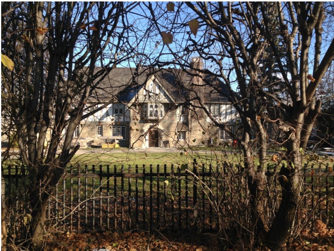
13. Pearce House, view from Kingsway Crescent of the west elevation with the iron fence and substantial planting along the edge of the property. (Heritage Preservation Services [HPS], 2018)
