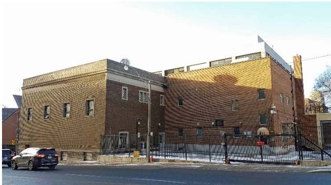
4b. East (left) and north elevations (with Eglinton Control Centre on the right)
