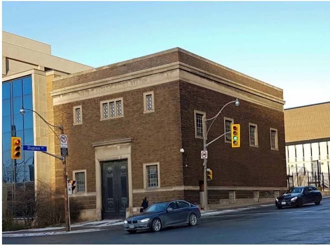
4a. Principal (left) and east side elevations
