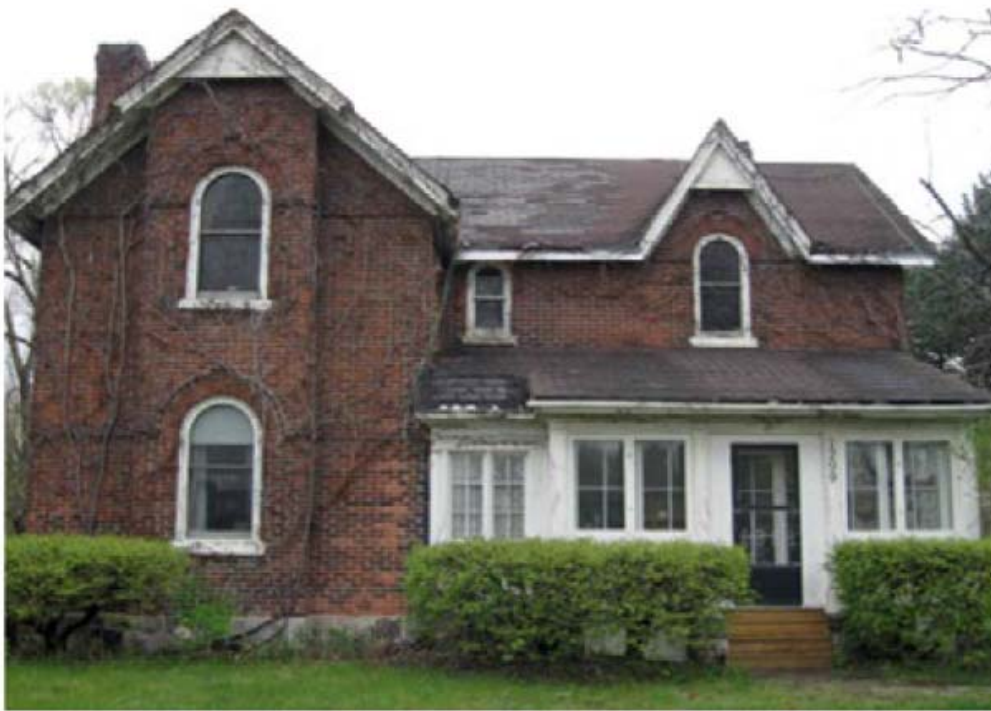
View (facing east) of the existing property's primary west elevation, including the one-storey sunroom.
