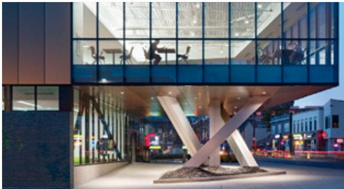
Architectural Features can contribute to the public realm. Northside Library, Columbus, Ohio, US.
