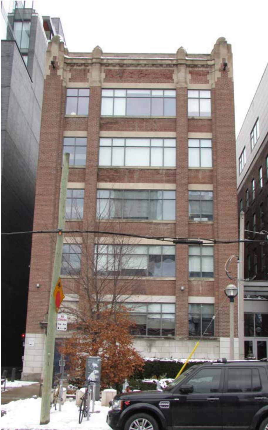
488 Wellington Street West – South/primary façade
