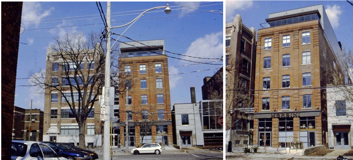
5d. and 5e. archival photographs, 2001, showing the 1990s rooftop addition to the 1907 warehouse (right) and the ground-level link between the two buildings
