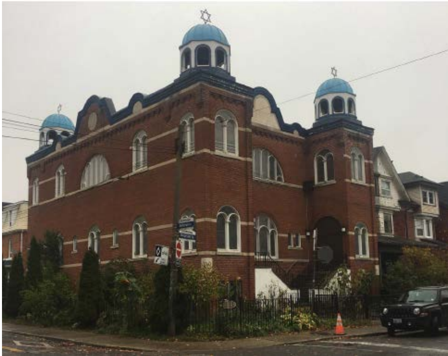
Kiever Synagogue, south and west elevations, view from the west side of Bellevue Avenue.
