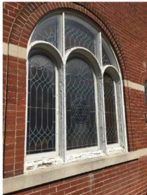
Cupola (left) and south elevation window showing typical signs of deterioration.
