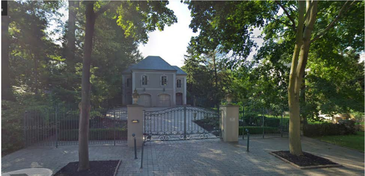
Contextual view (looking south) of the existing house to be demolished at 65 Binscarth Road
