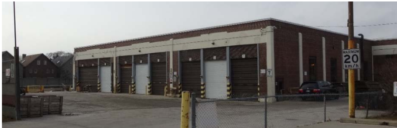
8c. south part of the east elevation
