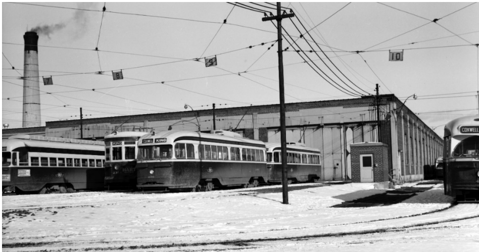
6b. 1959 view of the west elevation (left) from Coxwell Avenue
