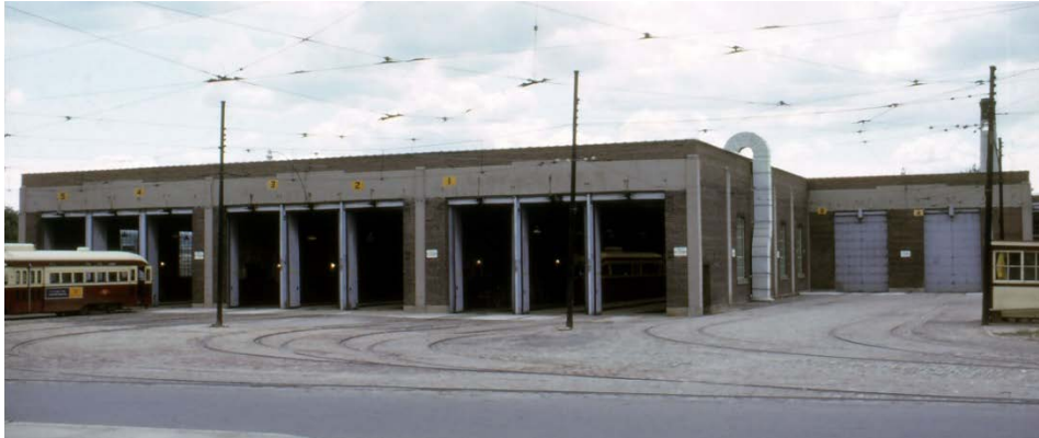
7a. 1964 view of the east elevation from Hillingdon Avenue
