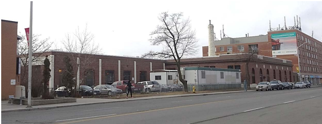
View from Danforth Avenue of the north end of the Danforth Carhouse (looking west to Coxwell Avenue)
