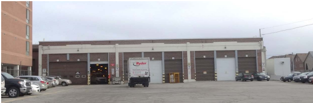
View from Coxwell Avenue of the west end of the complex (part)
