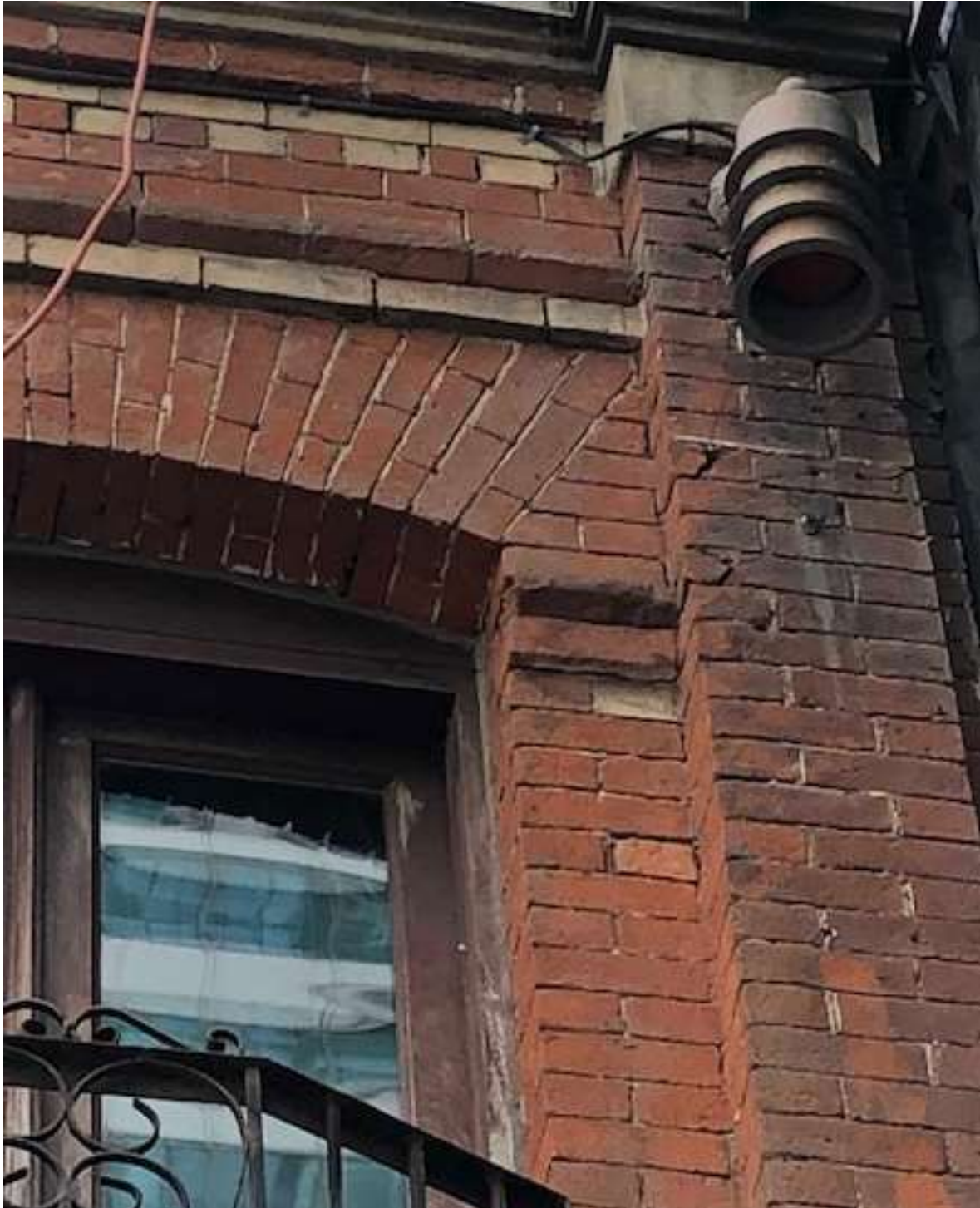
Masonry detail showing sandblasted bricks and mortar deterioration
