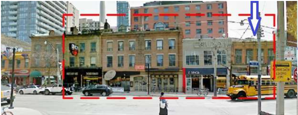
Existing King Street frontage of development with subject property (blue arrow)
