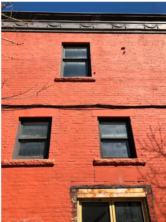
21a. (left) 348 Yonge Street - south elevation, detail showing pressed metal frieze and cornice, bricks, lintel and sills (HPS, 2019)
