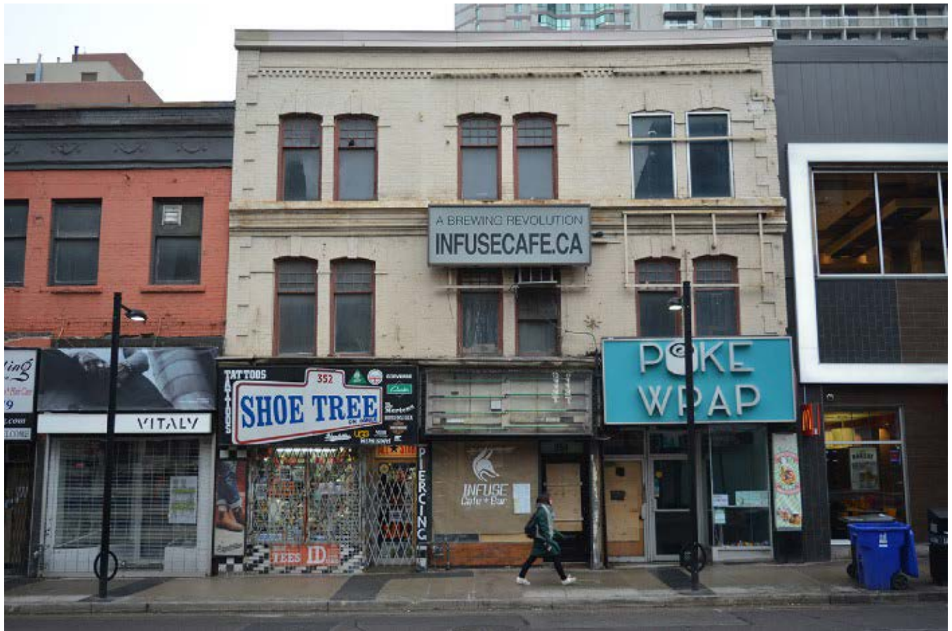
352 – 354 Yonge Street – east/front façade at Yonge Street
