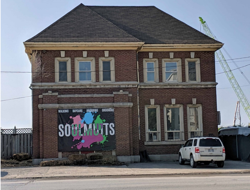
Above: principal (north) elevation, Fire Hall No. 30 (Heritage Preservation Services, July 2019); cover: aerial photograph, oriented with north on the top ( www.google.ca/maps )
