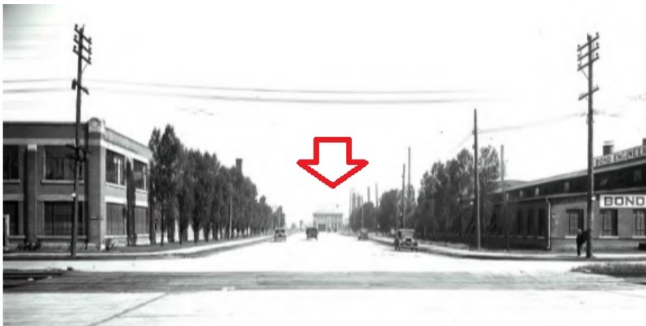
4c. Archival photograph, view south on Munition Street to Fire Hall No. 30, 1928
