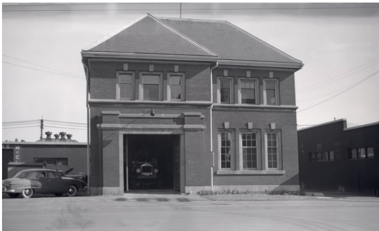
5c. Archival photograph, 1952, Fire Hall No. 30 with equipment bay
