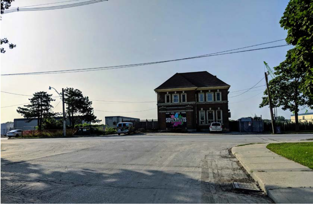
39 Commissioners Street from Munion Street showing north elevation
