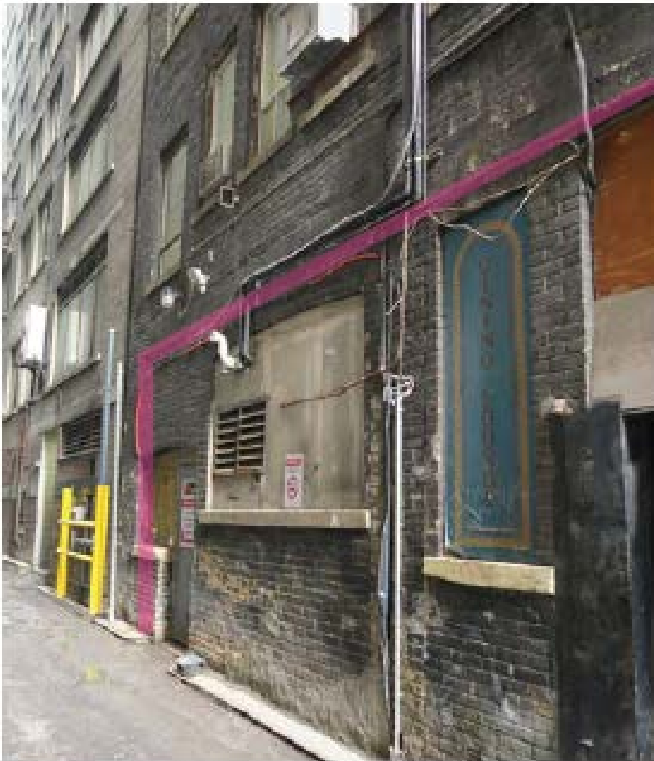
Rear (west) elevation of 56 Yonge from laneway; pink line denotes zone below concrete sill (ERA, 2019).
