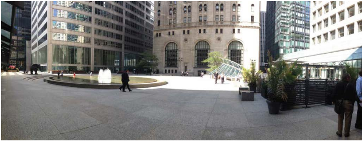
The Commerce Court North and West buildings as seen from within the courtyard (ERA Architects)
