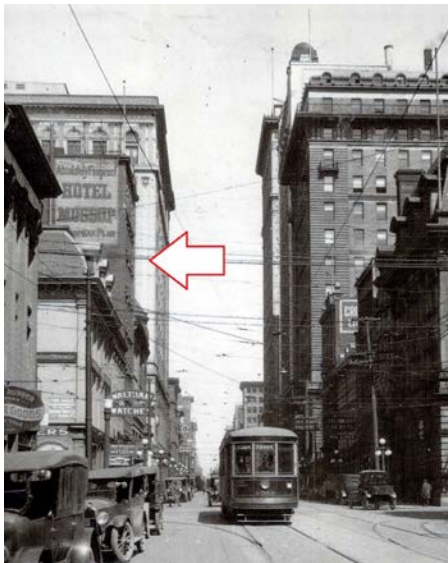
4a. principal (east) elevation, 1909; 4b. context looking north on Yonge Street, 1920s
