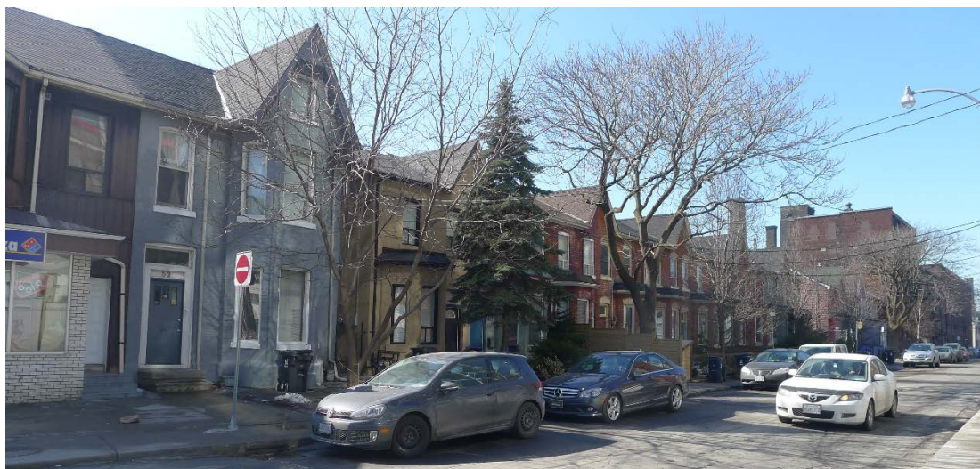
9. Niagara Street, 1885-1890: showing the consistent streetscape of housing built between 1885 and 1890 with the heritage-designated National Casket Company Factories at the far right. (Heritage Preservation Services, 2014)
