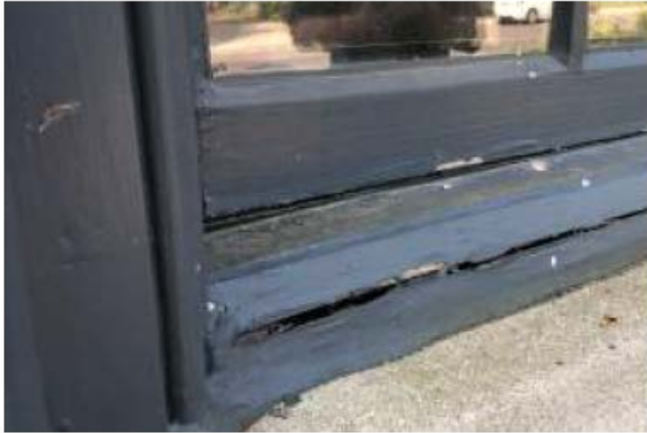
Heaved and split window sill
