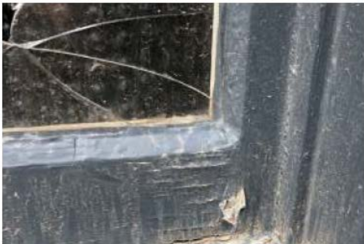
Broken glass pane & peeling paint
