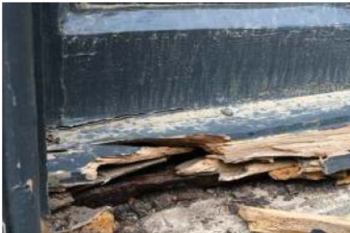
Broken sill, rusted substructure
