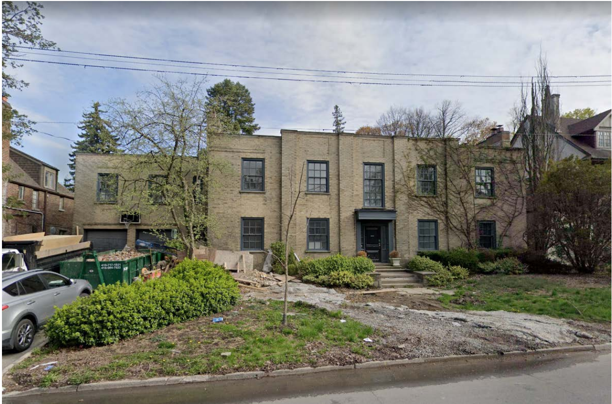
North elevation of subject property as viewed from the street
