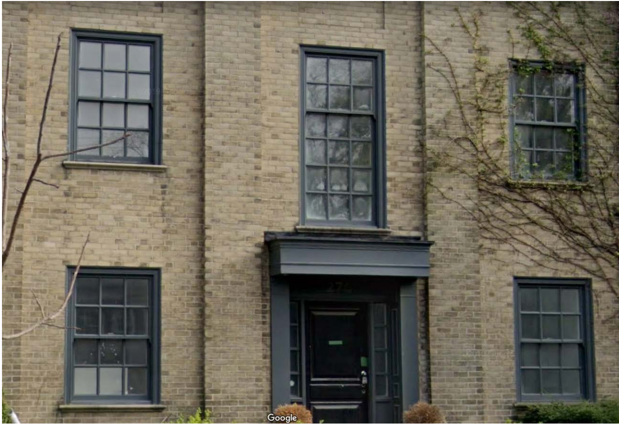
Detailed view of existing original windows on north facing elevation of the property
