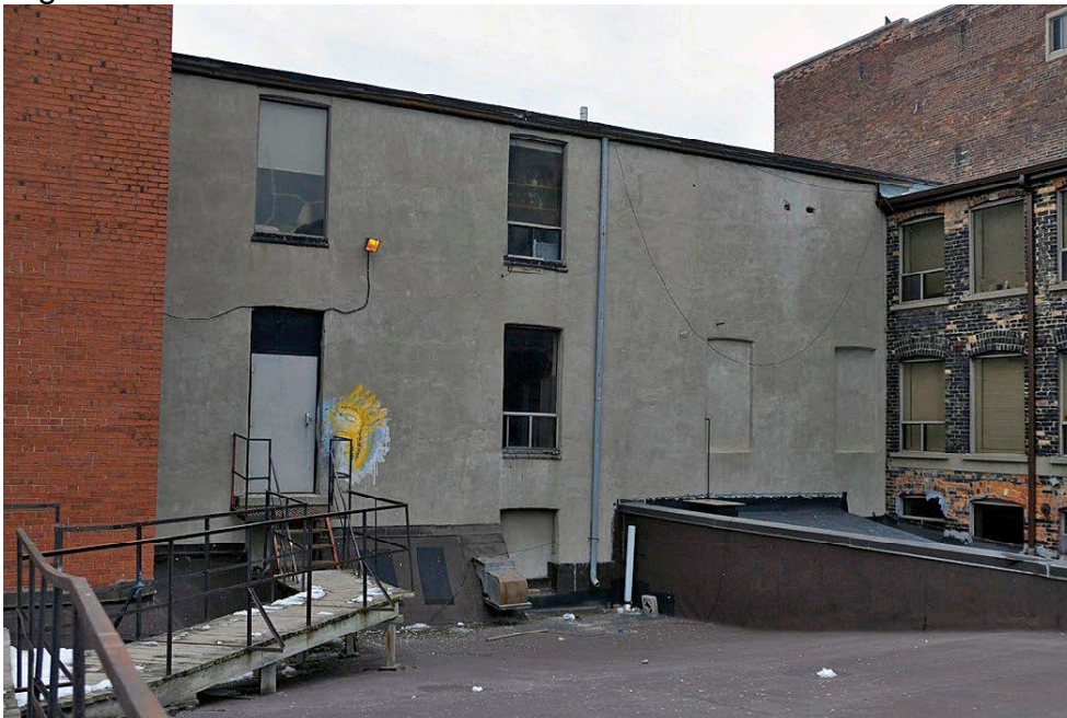
Rear elevation - 95-97 Niagara Street - Note, stucco cladding will be removed and brick will be repaired and repointed as needed.
