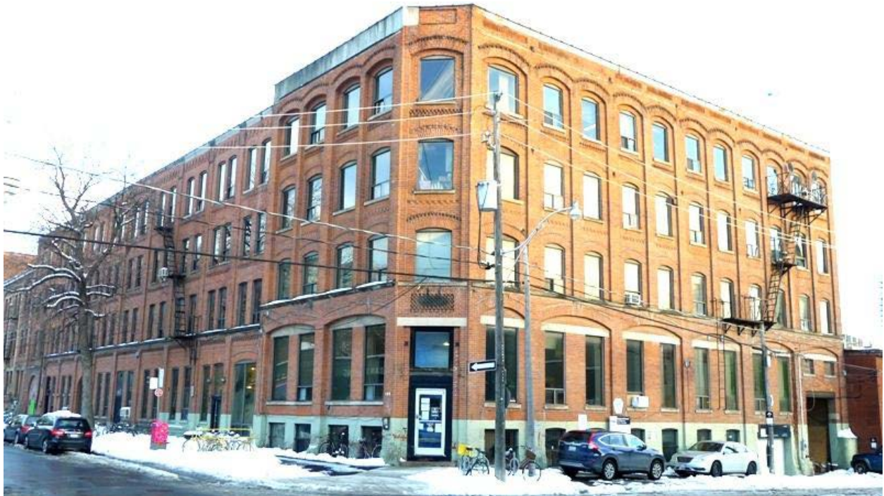
109 Niagara Street with Tecumseth Street frontage
