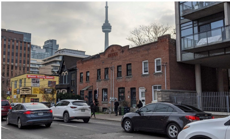
4e. 445-453 Adelaide Street West, context from west, 2019
