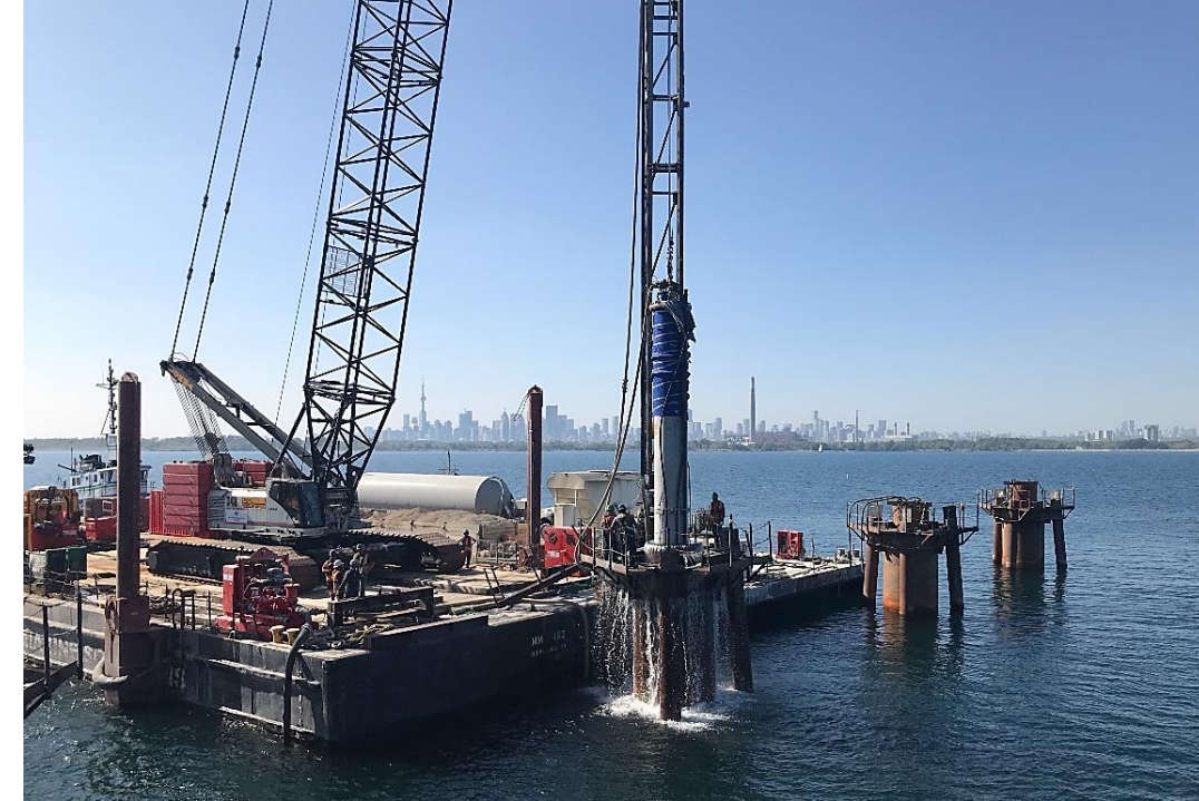
Ashbridges Bay Treatment Plant - New Outfall: Offshore platform in Lake Ontario. The new Outfall will improve capacity and better convey effluent from the Plant to Lake Ontario. Outfall is tunneled 85 meters deep beneath the lakebed, 3.5 km long; 50 risers to disperse treated and disinfected effluent to Lake Ontario.
