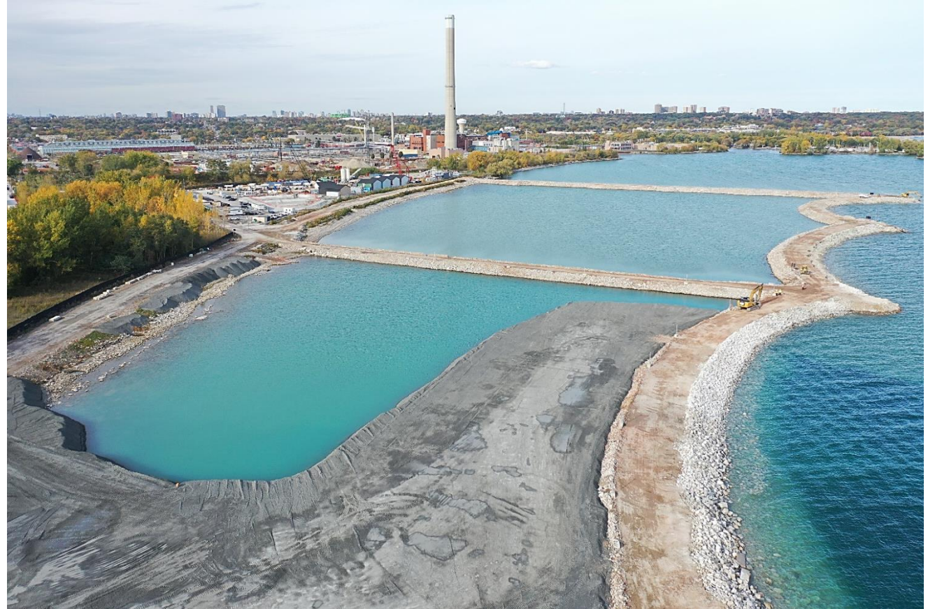
Ashbridges Bay Landform Project: Joint initiative between City of Toronto and TRCA. This project will provide erosion and sediment control to improve passage for boats, eliminating the need for regular dredging in the Coatsworth Cut area of Ashbridges Bay. It will also be the site of the high-rate treatment facility and a stormwater treatment wetland. The high-rate treatment facility is designed specifically to provide treatment of combined sewer overflows intercepted by the new Don River and Central Waterfront tunnel system.
