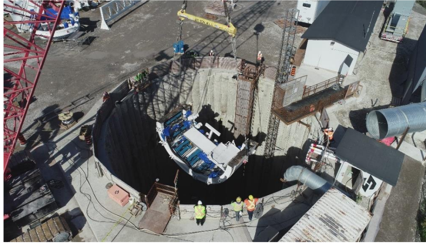
Don River & Central Waterfront Project - Ashbridges Bay Treatment Plant New Outfall: Above, tunnel boring machine being lowered into the shaft. The new outfall will improve capacity and better convey effluent from the Plant to Lake Ontario. Outfall is tunneled 85 meters deep beneath the lakebed, 3.5 km long; 50 risers to disperse treated and disinfected effluent to Lake Ontario. (Right: outfall tunnel entrance.)
