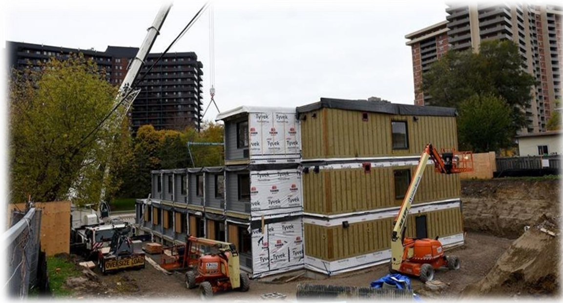
Construction progress as of October 28, 2020
