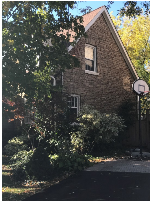
10 and 11. Current photographs detailing the fine craftsmanship of the stonework on all three cottages with the stone (allegedly locally sourced from Mimico Creek) being used on all four elevations and decorative detailing employed for the lintels of all openings in the form of stone voussoirs and keystones. (Heritage Planning, 2020)
