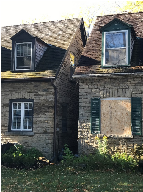
10 and 11. Current photographs detailing the fine craftsmanship of the stonework on all three cottages with the stone (allegedly locally sourced from Mimico Creek) being used on all four elevations and decorative detailing employed for the lintels of all openings in the form of stone voussoirs and keystones. (Heritage Planning, 2020)
