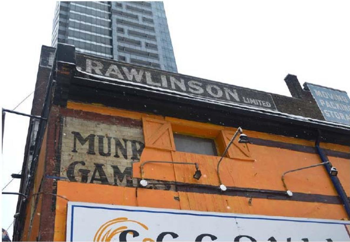
Close-up of the top of the south (side) wall showing a portion of the "Munro Games" sign, which was likely applied in the 1950s when the building was occupied by this company. The sign is in good condition, albeit dirty. Bricks are in fair to good condition. The removal of the board which was hiding the sign (the board was itself a subsequent sign) did not appear to damage the bricks.
