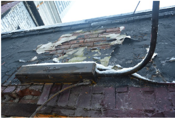
Top left: Close-up of the parapet. The peeling paint reveals cement parging. Removal of this parging will further damage the bricks. Mortar has eroded. Parapets typically require to be dismantled and reconstructed. Note the broken bricks above the window lintel (the lintel is metal).
