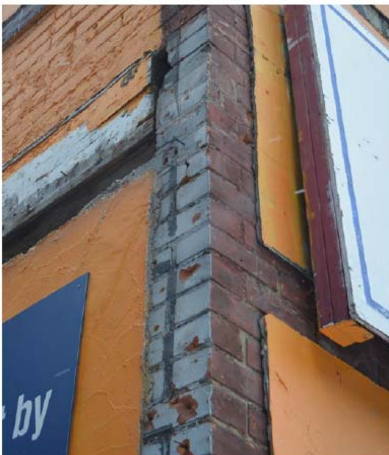
Close-up of corner of building. Note the damaged bricks following the removal of the wood trim. The trim was nailed directly on the bricks, thus damaging the surface.
