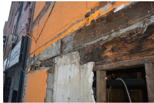
Top right: Close-up of a window opening. Note the concrete masonry units (on the right side and the bottom portion of the window). Bricks above the window are bulging outwards and some are broken (red arrow). Mortar has eroded heavily.
