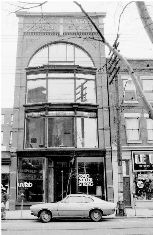
8c. Archival photo of the principal (south) elevation at 98 Queen Street East (Toronto Historical Board, 1973)
