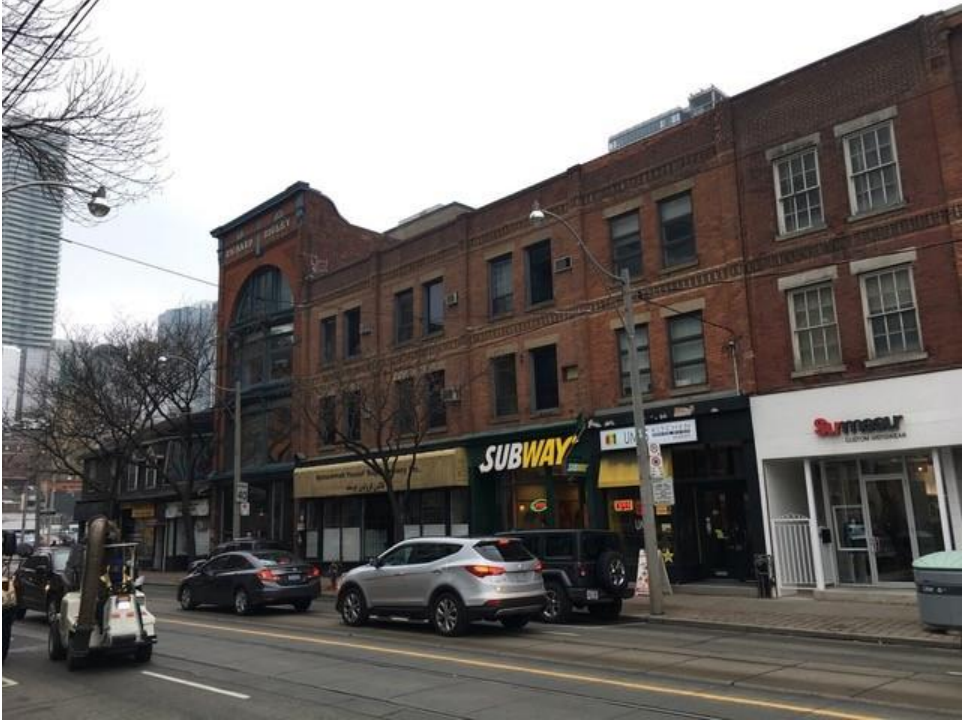
South facades of site facing Queen Street
