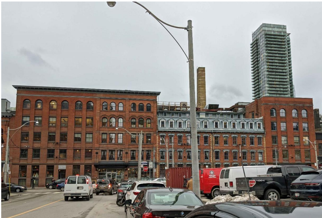
10. Properties on the south side of Queen Street at Mutual Street
