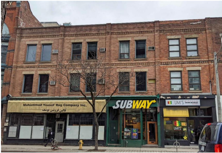
9i. Photograph of the properties at 100, 102 and 104 Queen Street East including 106 Queen Street East at the far right. (HP, 2019)
