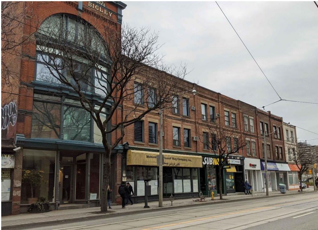
9g. Photograph showing the Richard Bigley Building and the properties at 100-104 Queen Street East, which are part of a row extending from 100-112 Queen Street East (HP, 2019)
