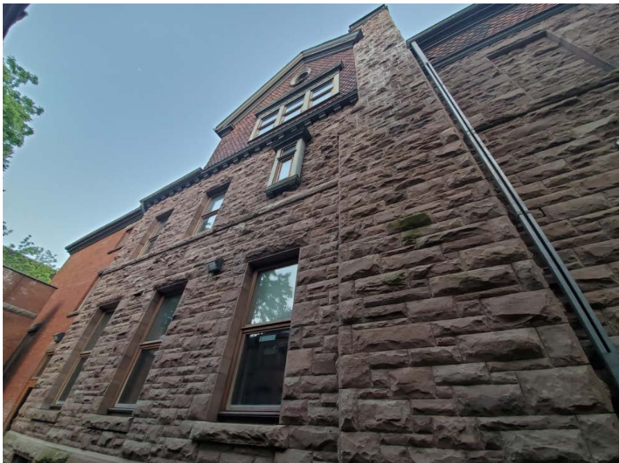
23. Detail of the side (north) elevation of the Alexander McArthur House (Heritage Planning [HP] Photo 2020)
