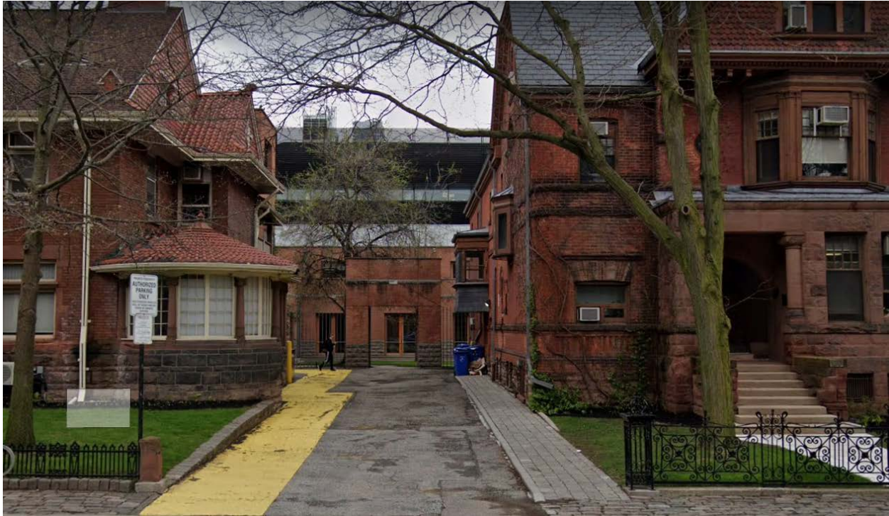
29. Detail of an entrance to the Peter F. Bronfman Courtyard from St George Street between 121 (right) and 123 (left) St George Street (Google Streetview 2019)
