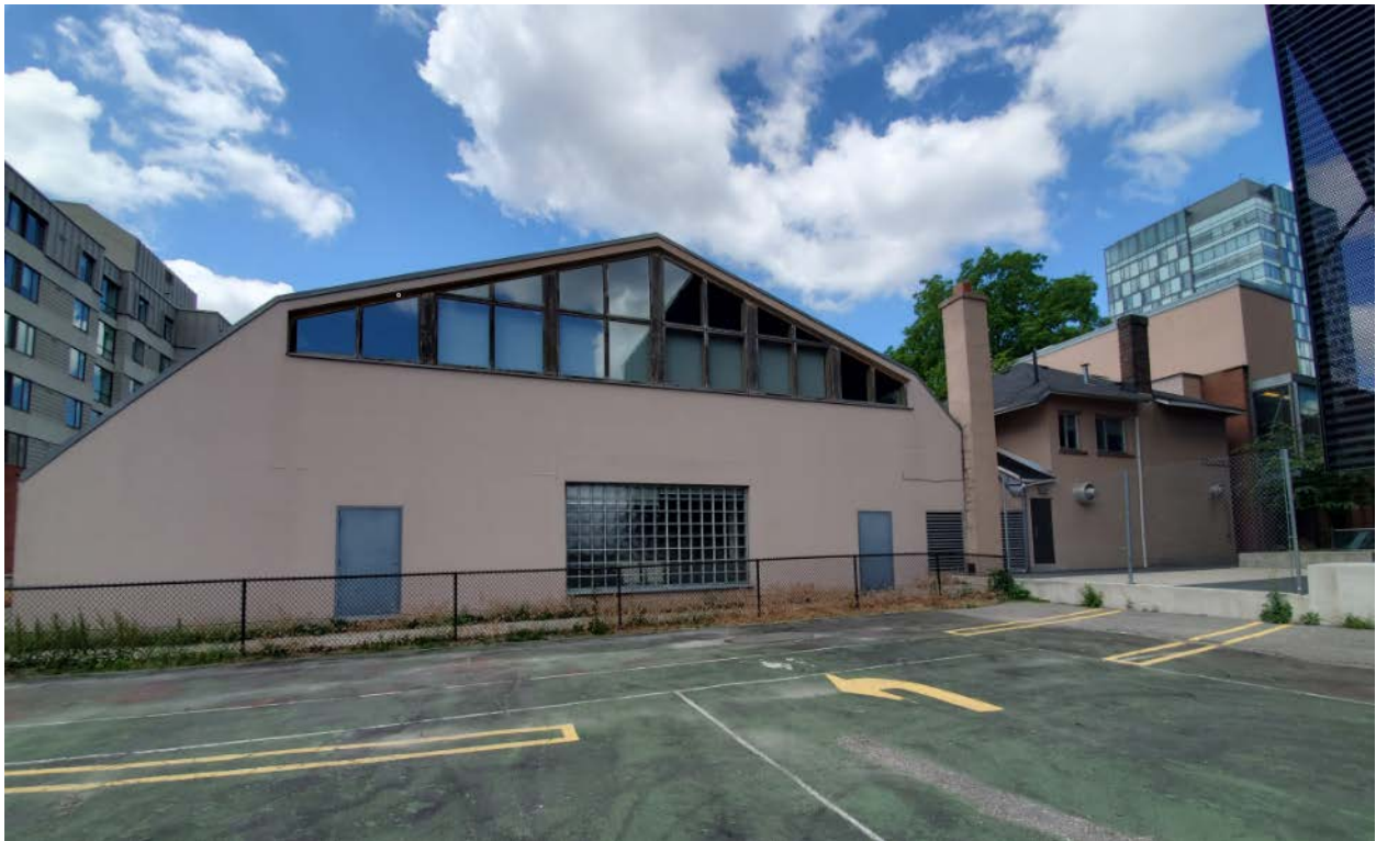
24. Detail of the rear (east) elevation showing the former Drill Hall (left) and the Margaret Fletcher House (right) (Heritage Planning [HP] Photo 2020)
